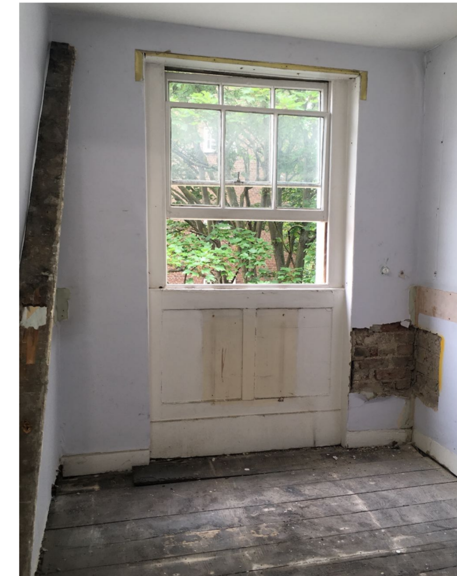
IMG_6982 Third Floor TOR304-Office
