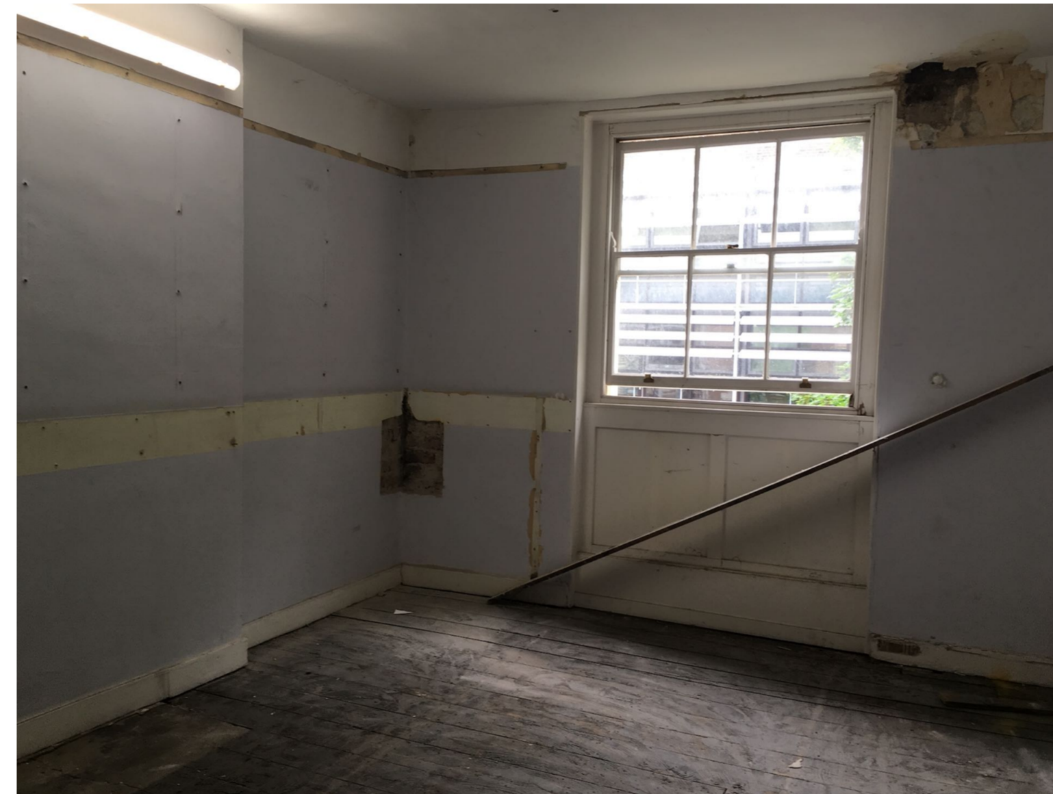
IMG_6983 Third Floor TOR303-Office
