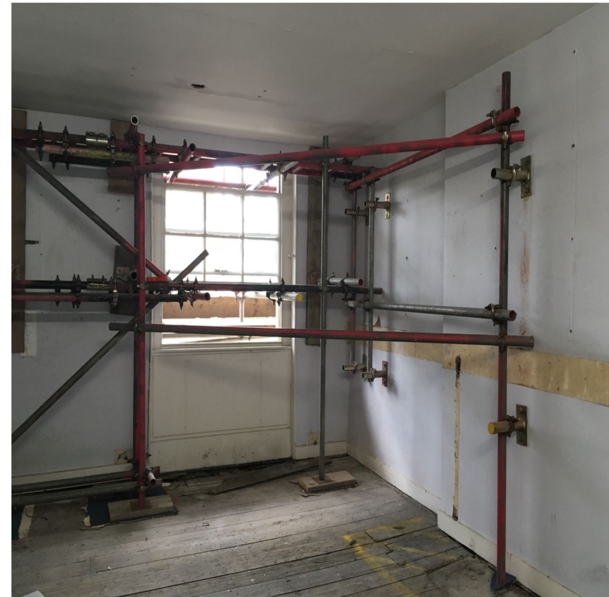
IMG_6984 Third Floor TOR302-Office
