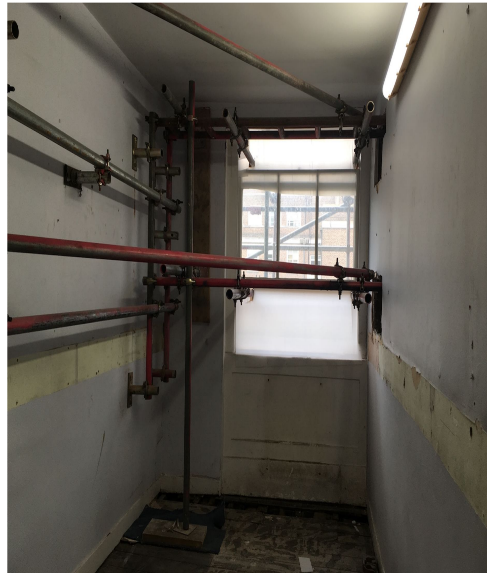
IMG_6985 Third Floor TOR301-Office
