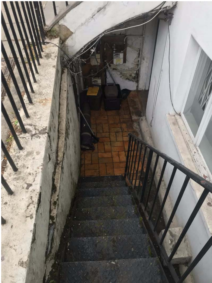
Photograph of 52 Delancey Street from top of stairs to lower ground
