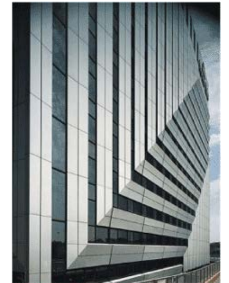
Anodised aluminium can be used to create modern advanced designs - here on a landmark building in Paris-La-Défense constructed over 25 years ago
