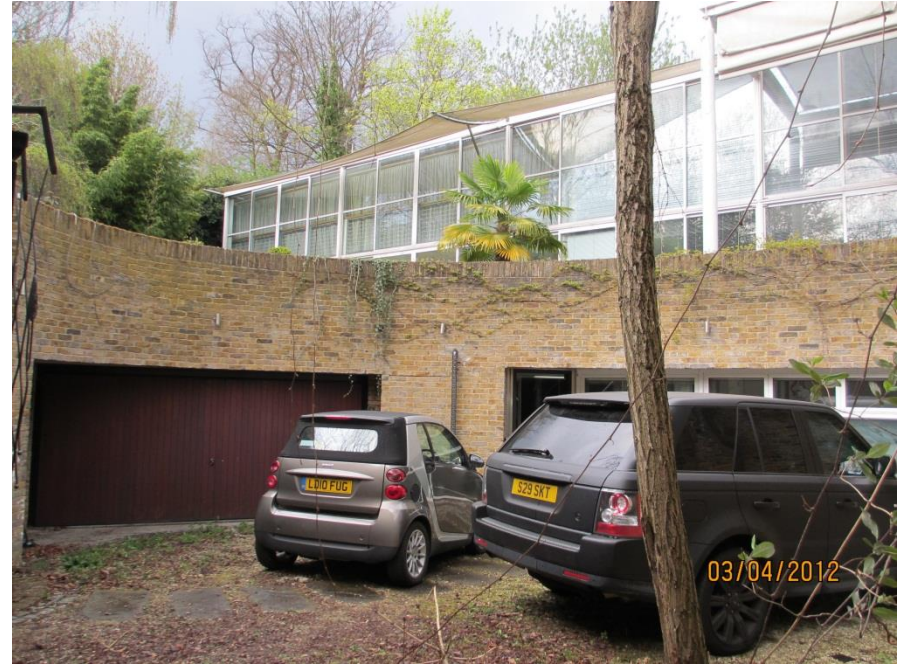
Photo 6: View Of Existing House and Garage
