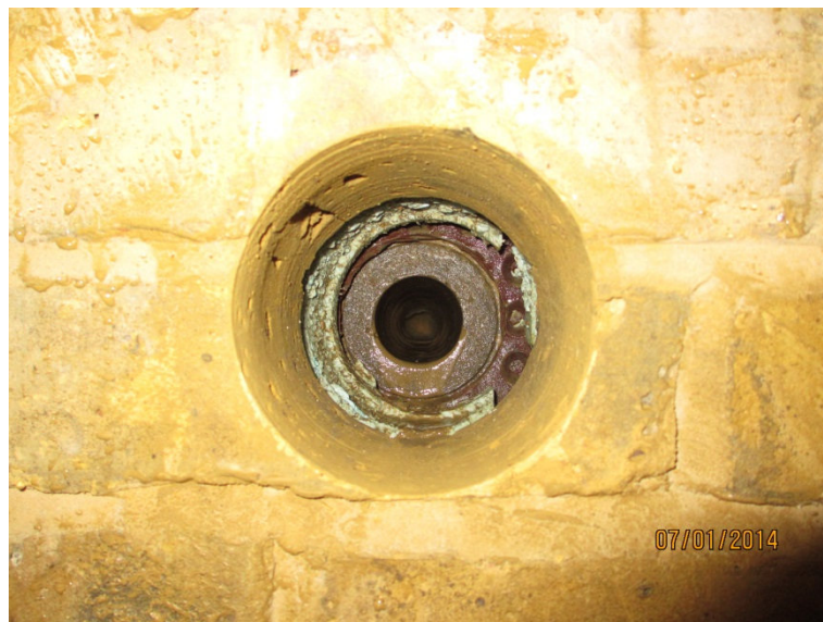
Photo 01 – Typical Core through Existing Wall
