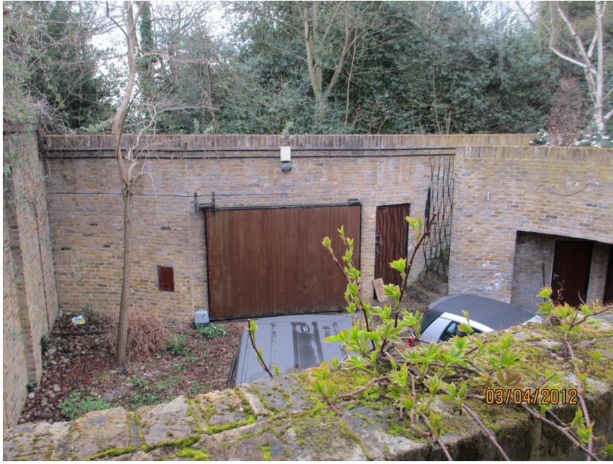
Photo 7: View Of Existing Entrance Onto Branch Hill
