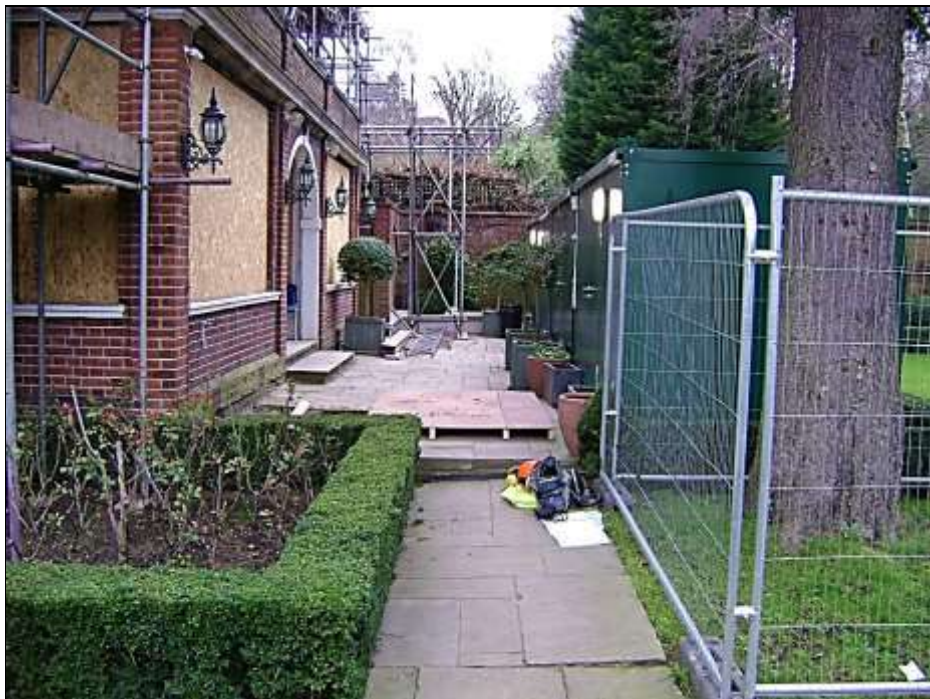
Photograph 2 – Looking down the side of the building and the location of the proposed single storey extension. The stem of the Cedar tree to the right of photograph.
