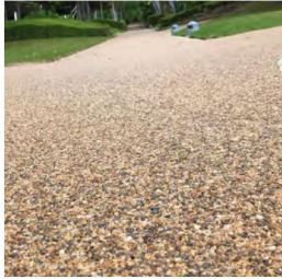
BARLEY BEACH PERMEABLE RESIN BOUND GRAVEL DRIVEWAY
