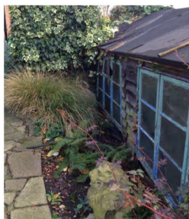
EXISTING CONDITION OF SHED. TO BE REPLACED WITH SAME STYLE SHED.
