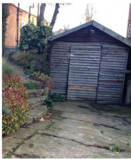
EXISTING CONCRETE DRIVEWAY, SHED AND STEPS
