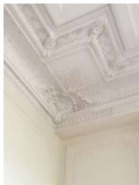
Cornice detail to Dining Room (4101) and Bedroom 1 (4109) Original fibrous plaster cornice with 4 elements; twin ogee and anthemion motif to ceiling, scotia and torus roll, finely decorated cavetto of interlocking flower and leaf pattern with torus roll and egg and dart to wall
