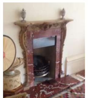
Timber moulding to opening, square jambs, brackets to shelf with central urn on frieze (Original) Cast iron pattern insert and slate hearth
