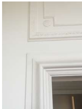
Original plaster moulding panels to walls in Dining Room (4101)
