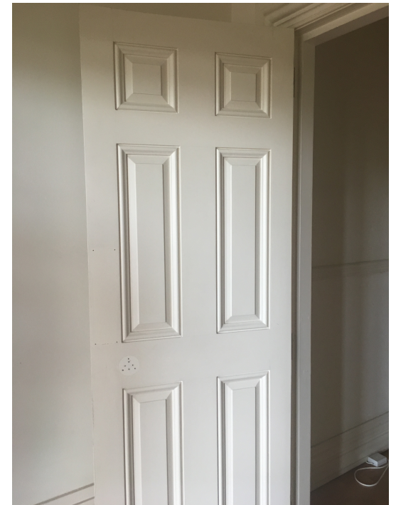
Existing Door Opening FD-02
