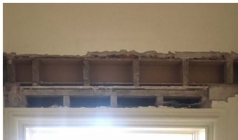
Exposed steel structure
