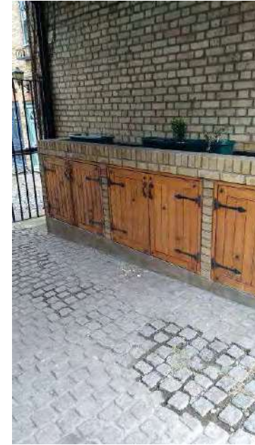
Bin store in archway.
