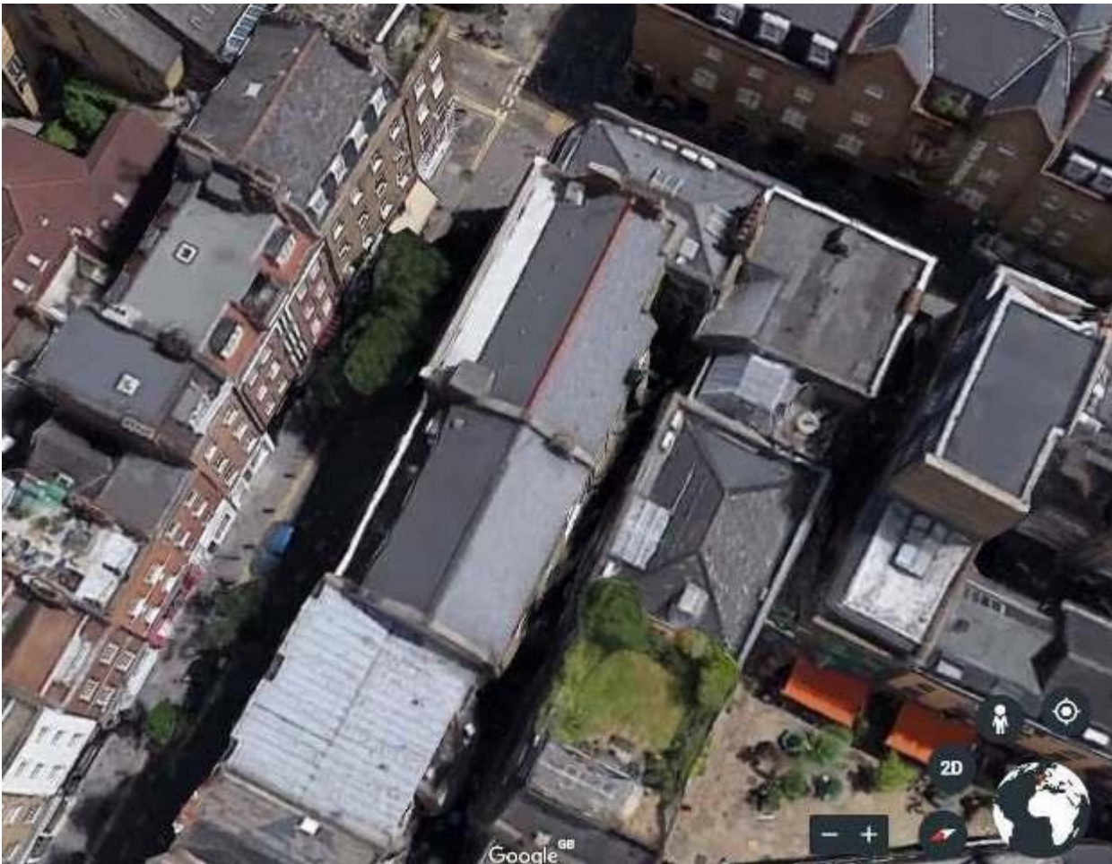
The roofs all appear original; however in the applicant's Heritage Statement the author has failed to investigate the roof timbers – see below re the CAS.
