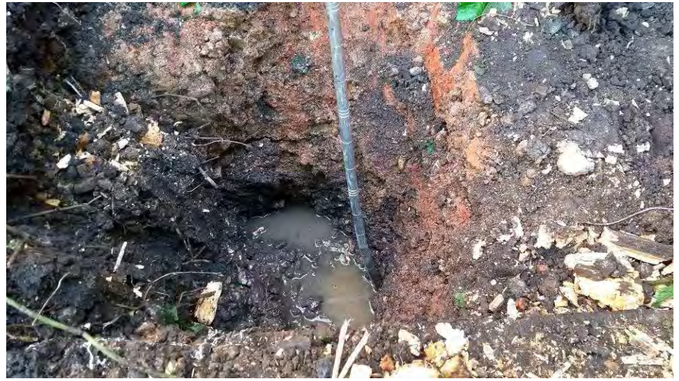
TP01 (foundation inspection pit).
