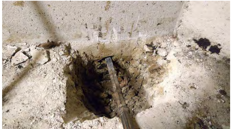
TP04 (foundation inspection pit).
