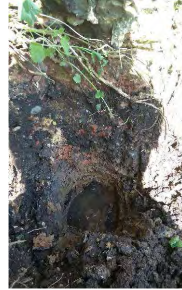
TPO3 (foundation inspection pit).
