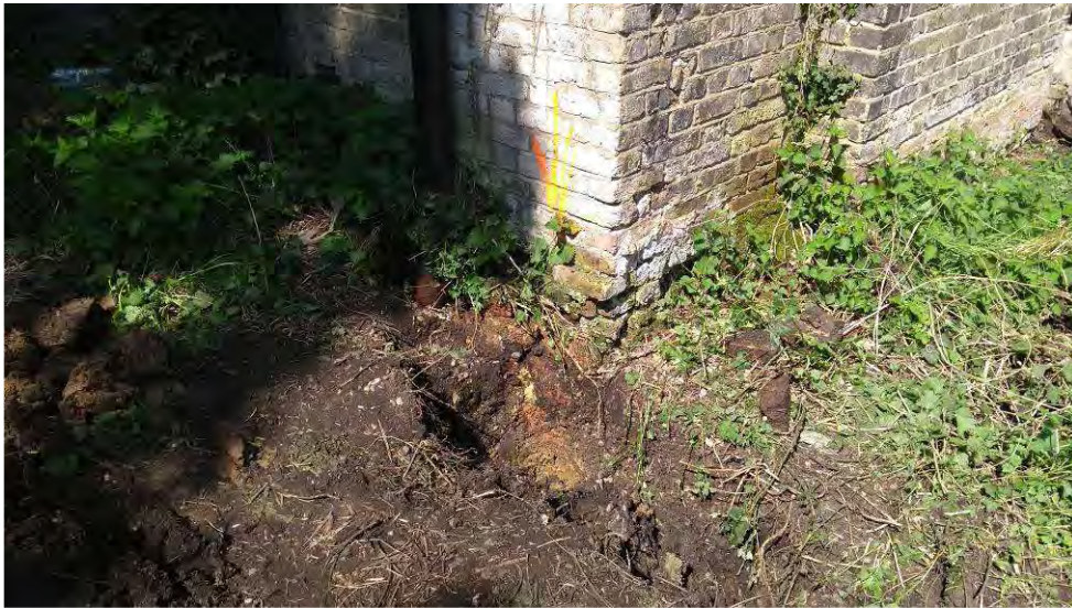
TPO3 (foundation inspection pit).
