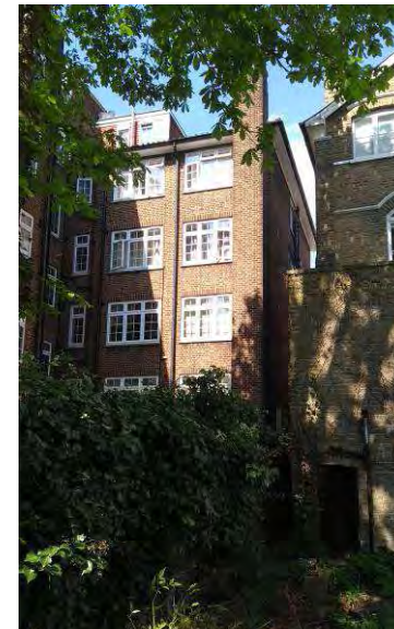
Neighbouring building (to west).
