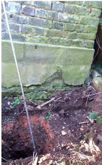
TP01 (foundation inspection pit).
