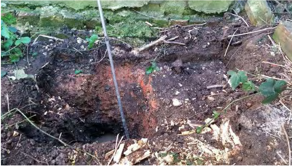
TP01 (foundation inspection pit).
