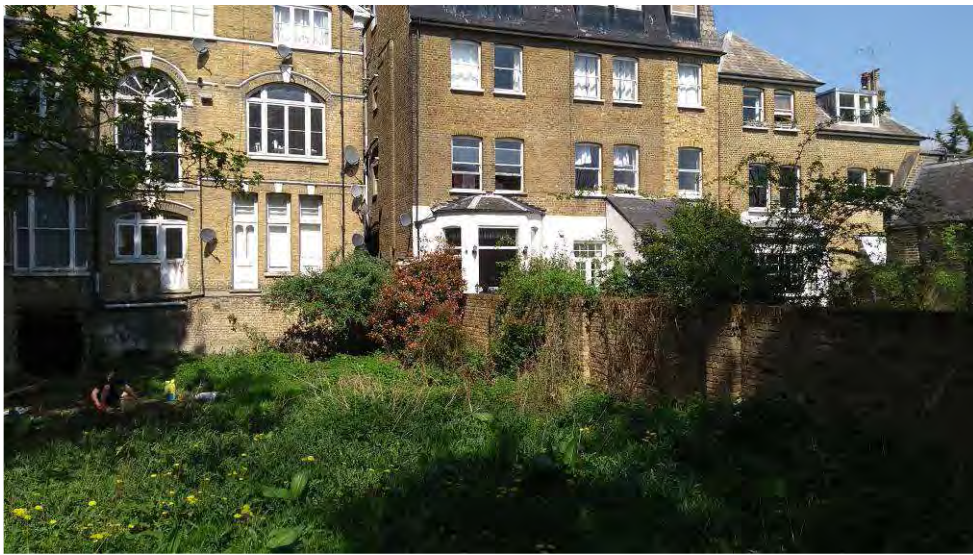
Adjacent building (to east).
