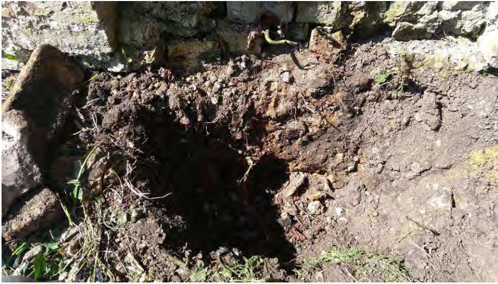
TPO2 (foundation inspection pit). Note roots.
