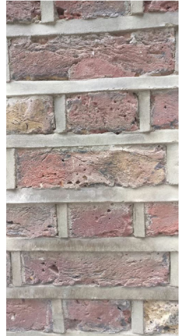
All external brick walls to be constructed using London Stock facia bricks to match Wells Court.
