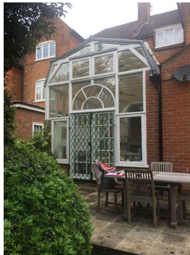
PHOTOGRAPH OF EXISTING CONSERVATORY
