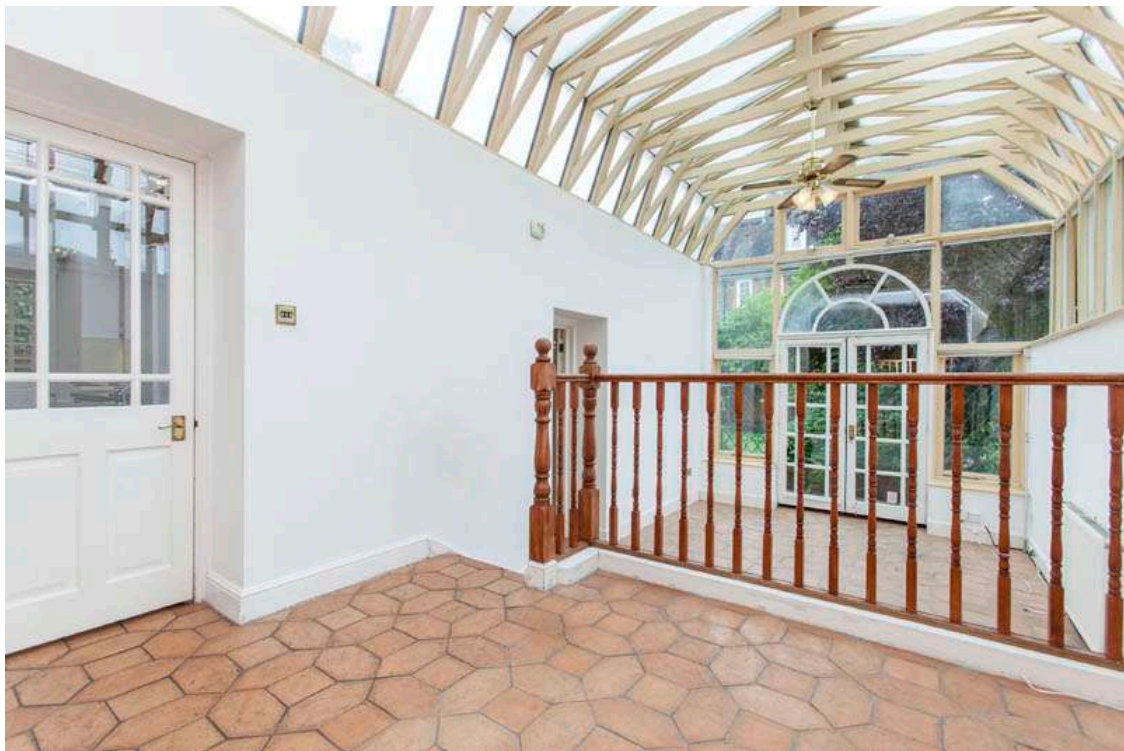
Existing internal view of the conservatory
