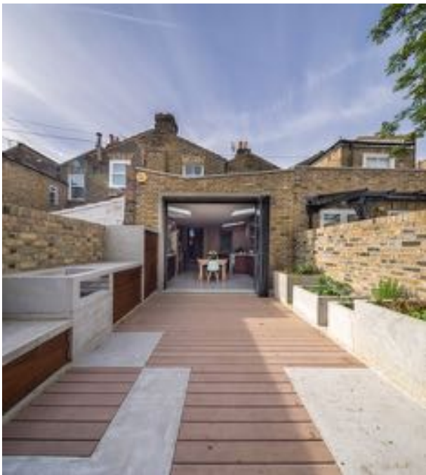
Figure 7: Extension in Tower Hamlets by Studio Gil
