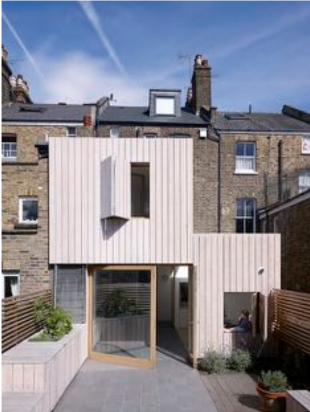
Figure 8: Extension in Hampstead Heath by Hayhurst and Co.
