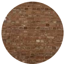
Existing Masonry Brick
