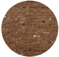
Existing Masonry Brick
