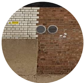
Existing Mixed Selection of Brickwork to Single Storey Extension.
