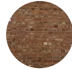
Existing Masonry Brick
