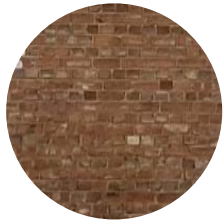
Existing Masonry Brick
