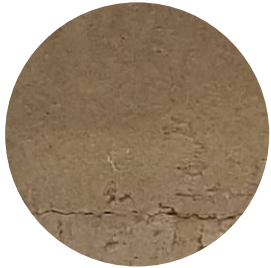
Existing Cementitious Render to Single Storey Extension
