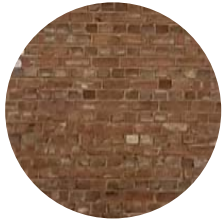
Existing Masonry Brick
