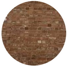
Existing Masonry Brick
