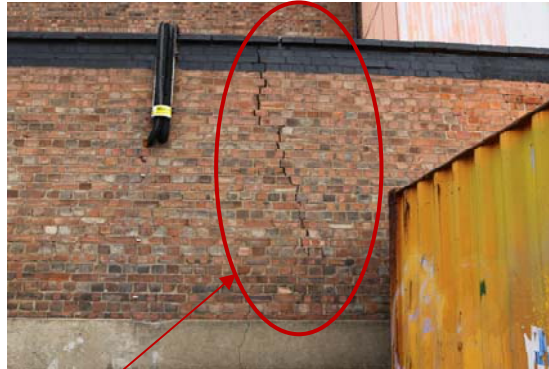
Significant Structural Cracking
