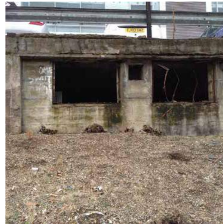
Vaults underlying southern corner of Phoenix Place
