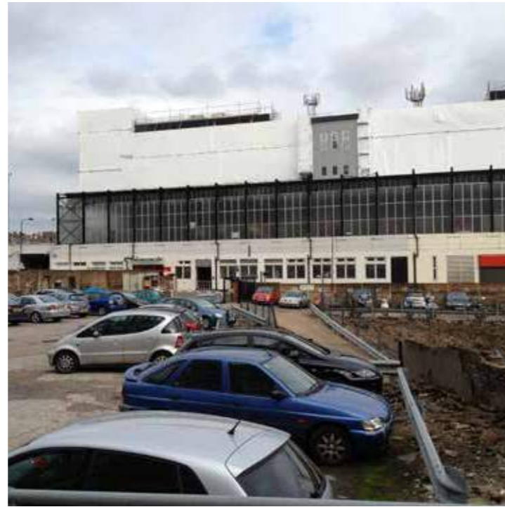
Phoenix Place looking north east
