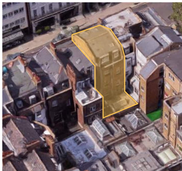
Figure 5: 10 Charlotte Street windows
