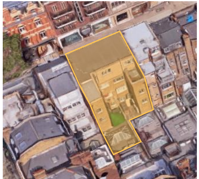
Figure 3: 3-4 Windmill Street windows
