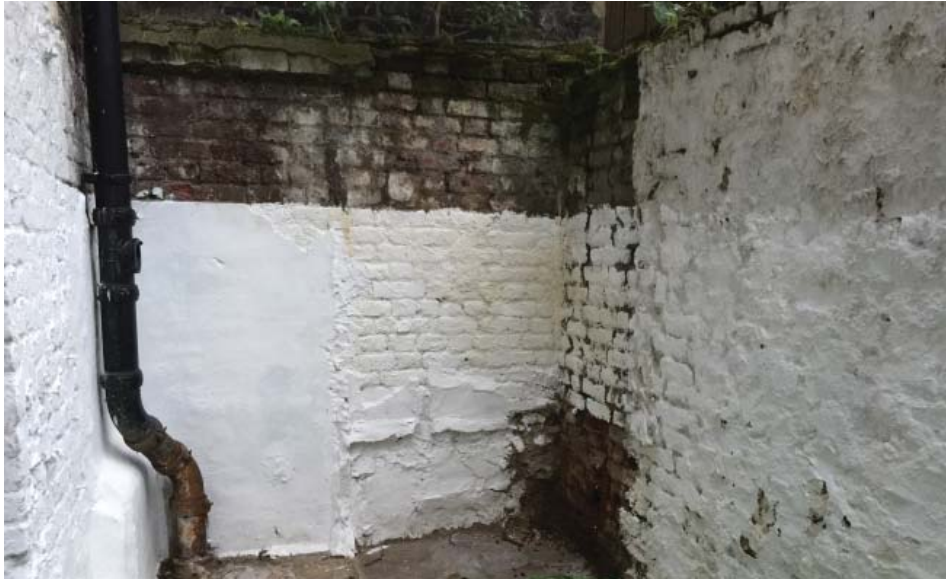
fig 6. view into existing rear courtyard
