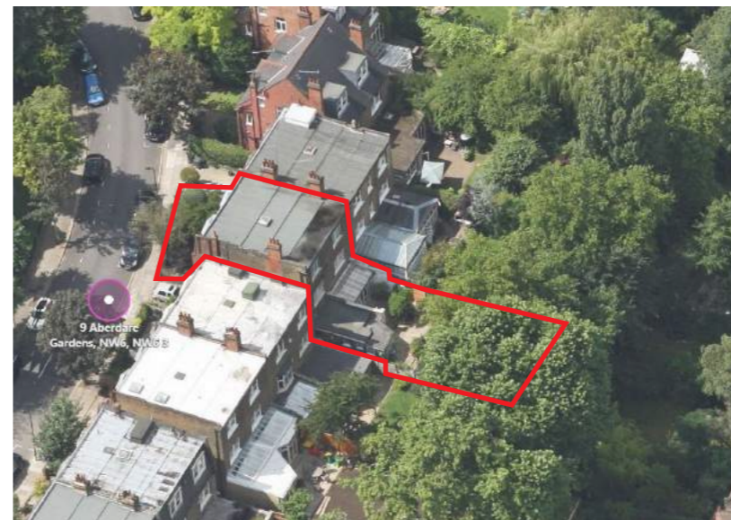
7 Aberdare Gardens and Surroundings Aerial View 02 (Site outlined in red)
