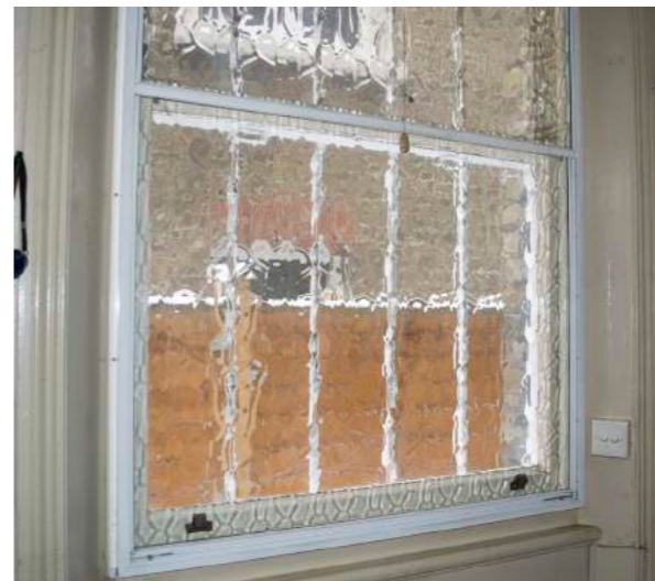
7 Aberdare Gardens Typical side elevation window & glazing bars
