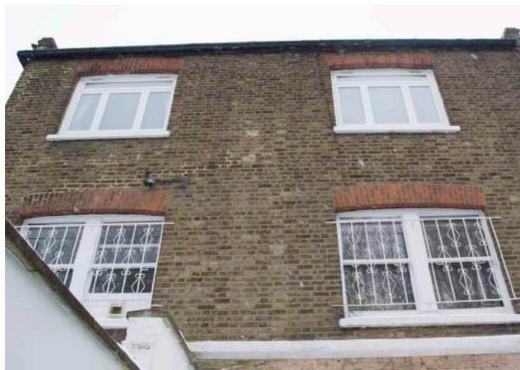
7 Aberdare Gardens Window bars to rear elevation
