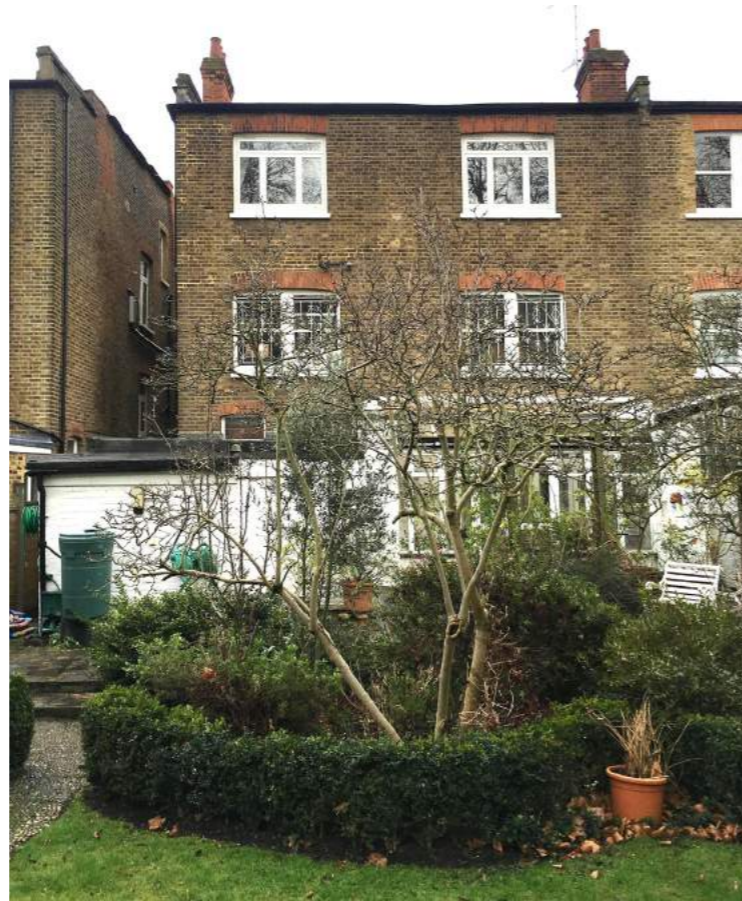
7 Aberdare Gardens Rear (North) Elevation
