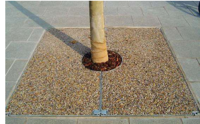
Recessed tree pits with resin bound gravel infill
