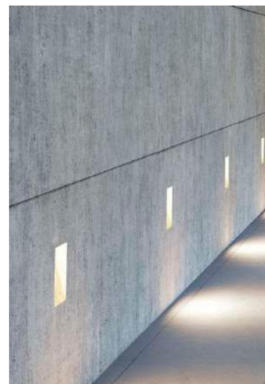
Inset lighting to concrete wall
