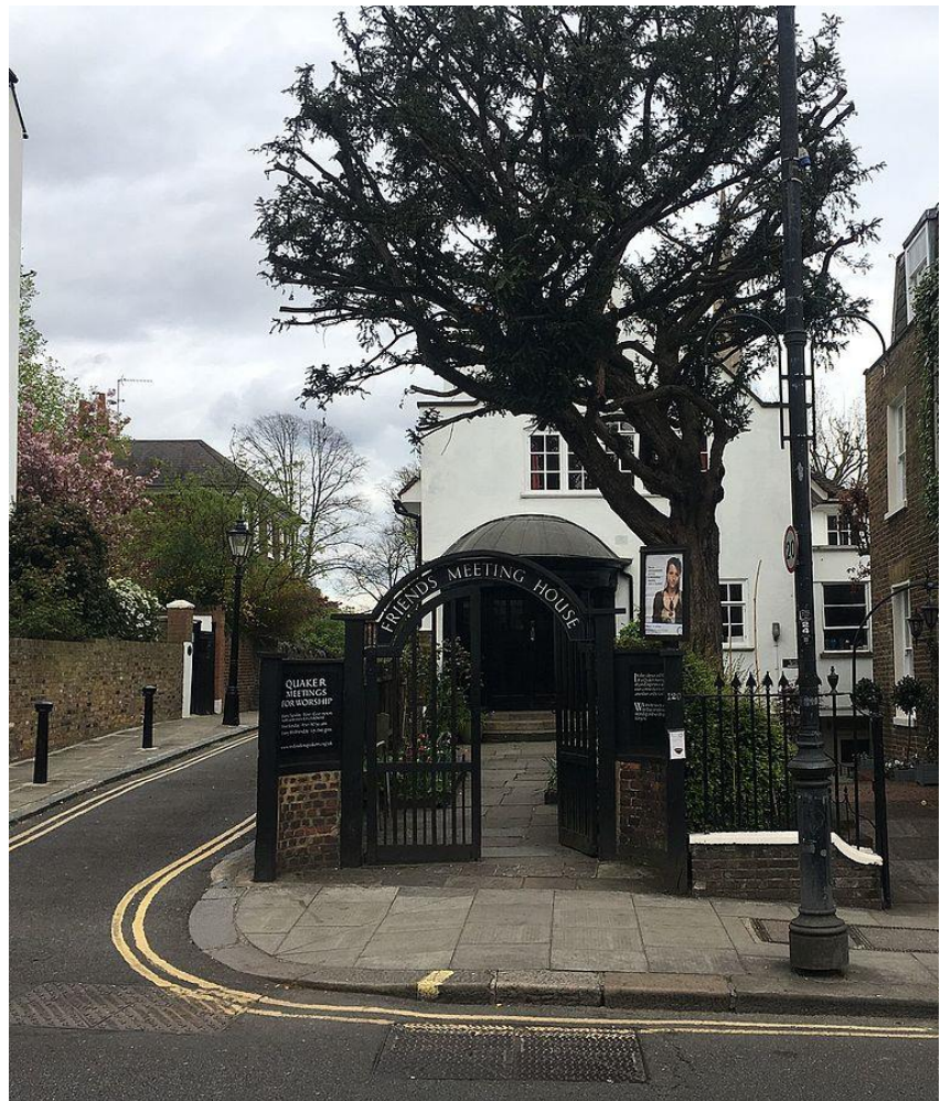
Fig.1 Main entrance to the building
