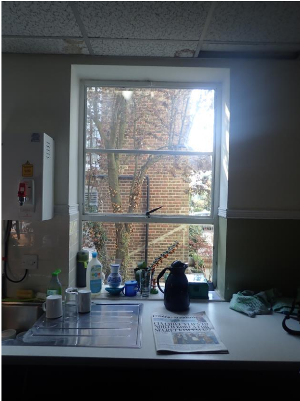
Fig 4 Side extension interior window
