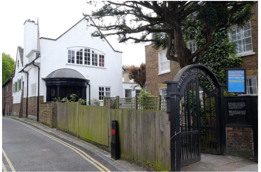
Fig.2. Building main elevation
