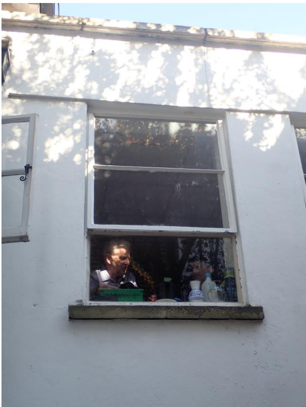
Fig 4 Side extension exterior window close-up
