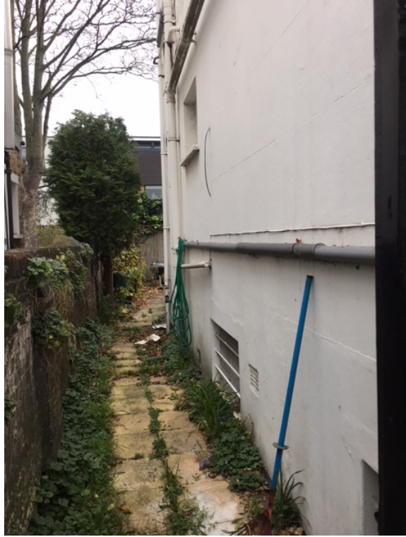
6. Side passageway of no. 99
