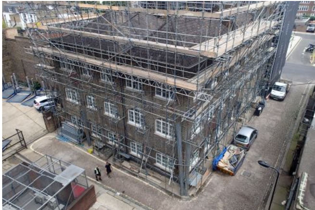
3 storey addition underway to 48-56 Bayham Place
