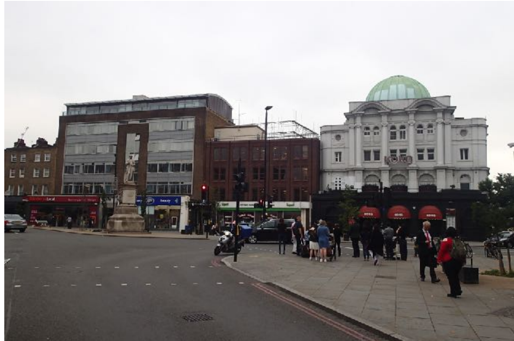
Existing building showing 3 storey addition to 48-56 Bayham Place
