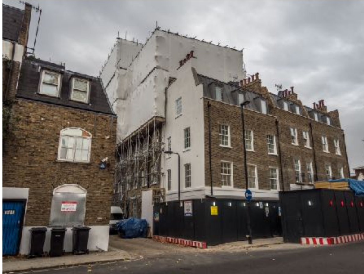
Entrance to Bayham Place showing extension to "Anders" building
