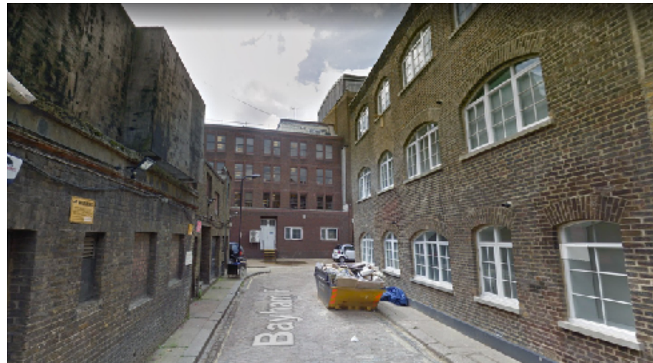
Long view of rear of site from Bayham Place
