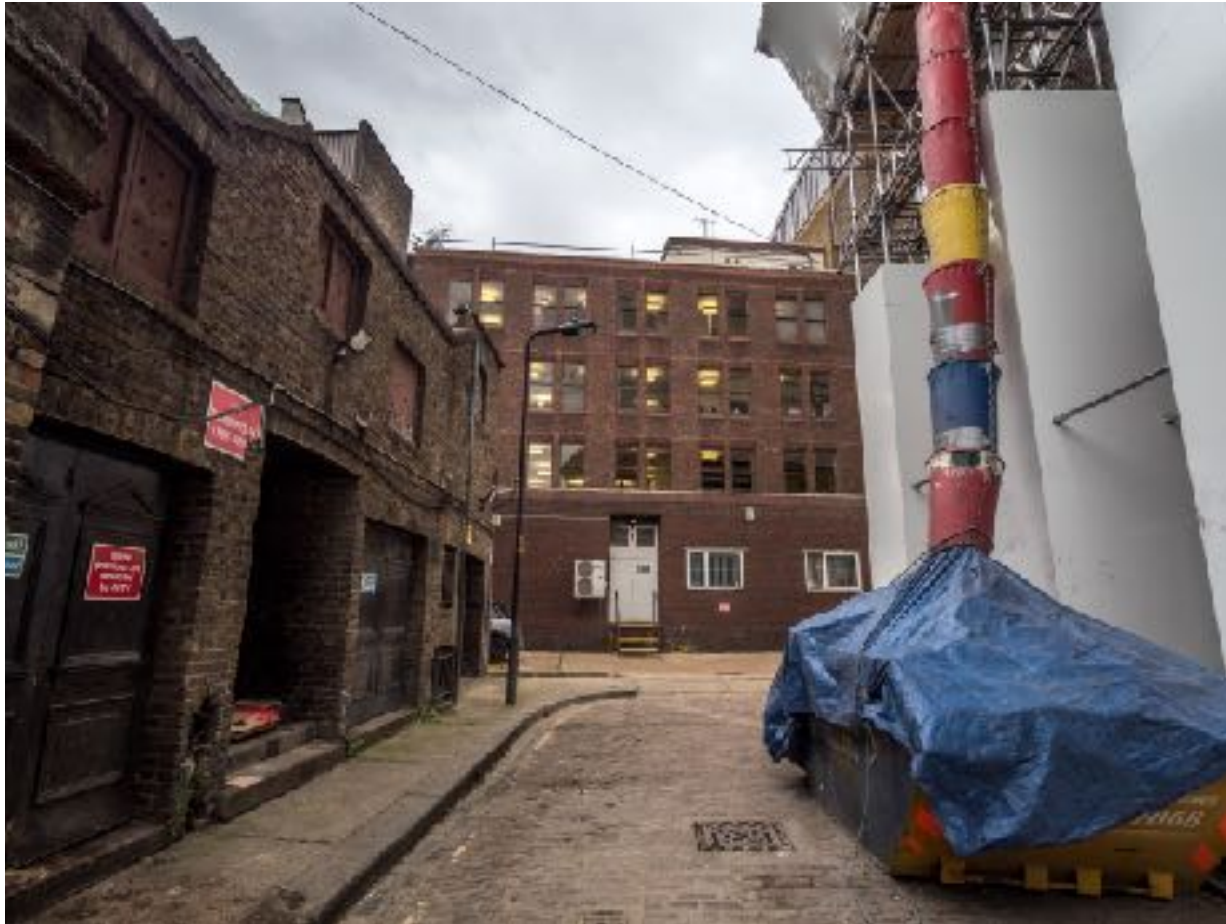
Rear of existing building from Bayham Place
