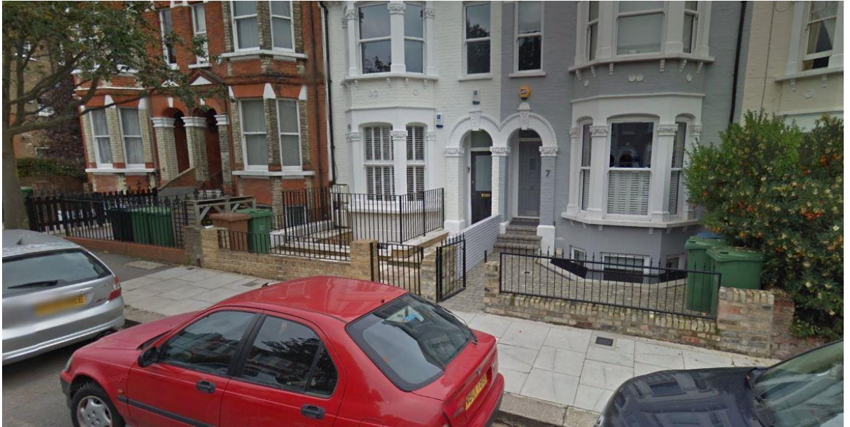
Light-well excavation at 3, 5 and 7 Kylemore Road, with bin storage area provided
