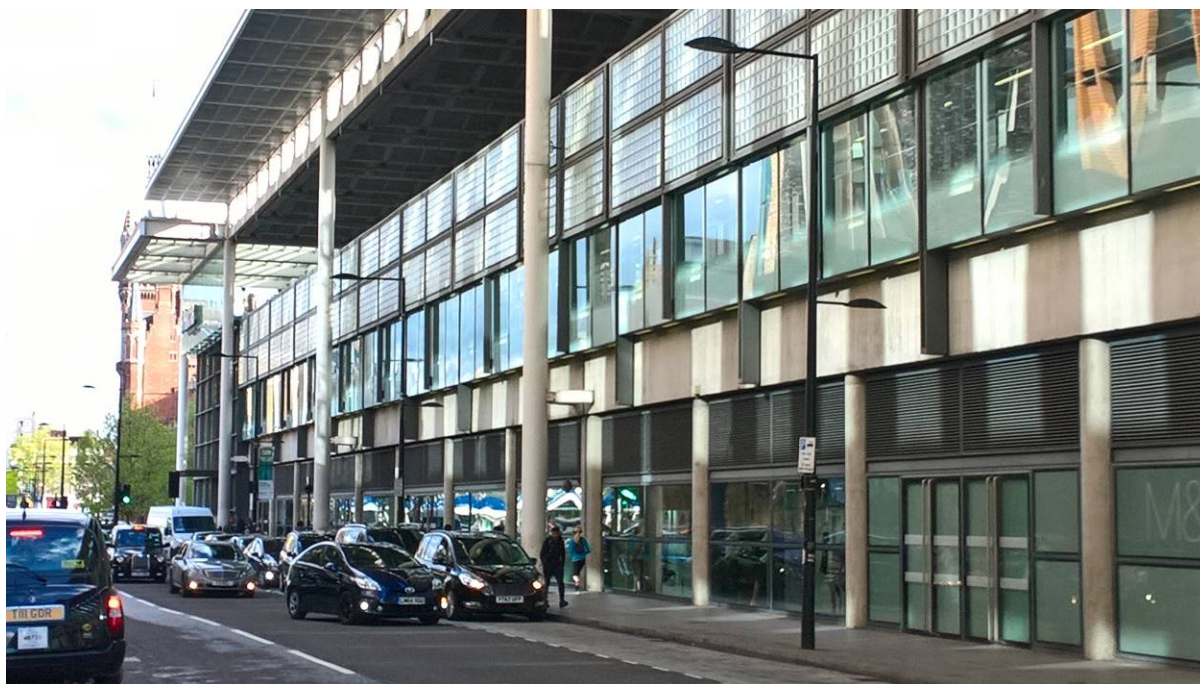
External elevation of St Pancras International (modern extension) on Pancras Rd.
