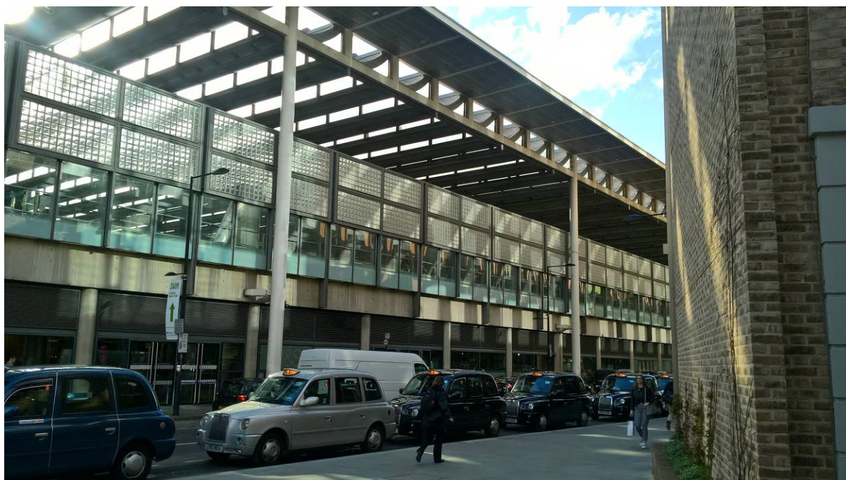
View onto affected external elevation of St Pancras International from the corner of the Stanley Buildings.
