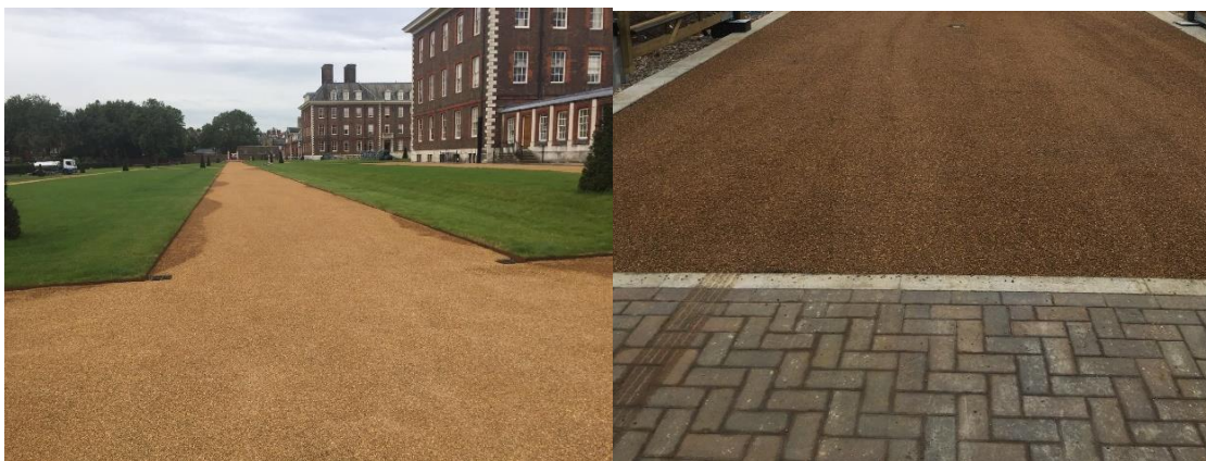
Figure 1: Asphalt and chip finish surface dressing (Source: Foster Contracting)
