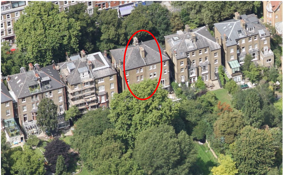
3. Aerial view from the rear
