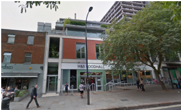
1) Front elevation of block from Pond Street
