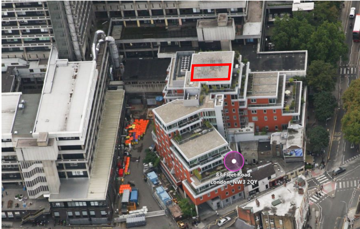
4) Aerial view of side elevation (proposed terrace area outlined in red)
