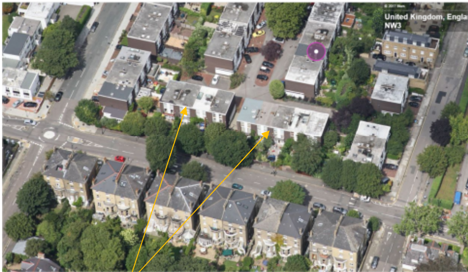
1. Aerial view of 24-32 Elliot Square with Elsworthy Conservation Area to the south
