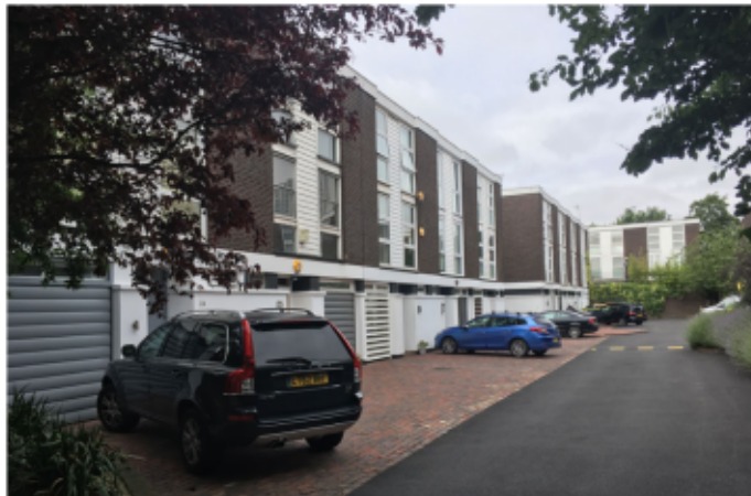
2. View of 24-32 Elliot Square from Elliot Square
