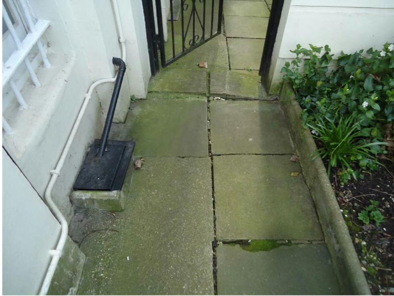
Photo 3 - Uneven paving leading into the lower ground floor
