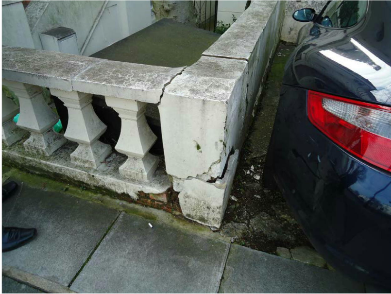
Photo 1 – Party fence wall
