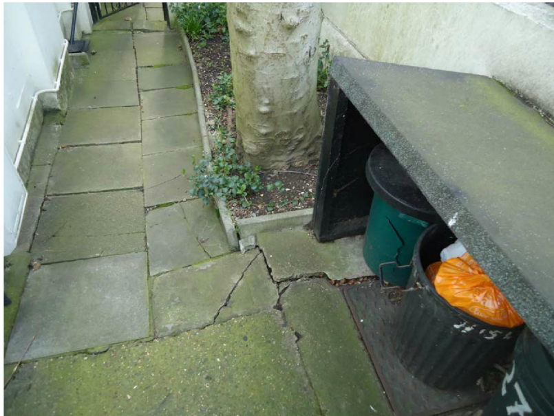
Photo 2 – Uneven paving leading into the lower ground floor
