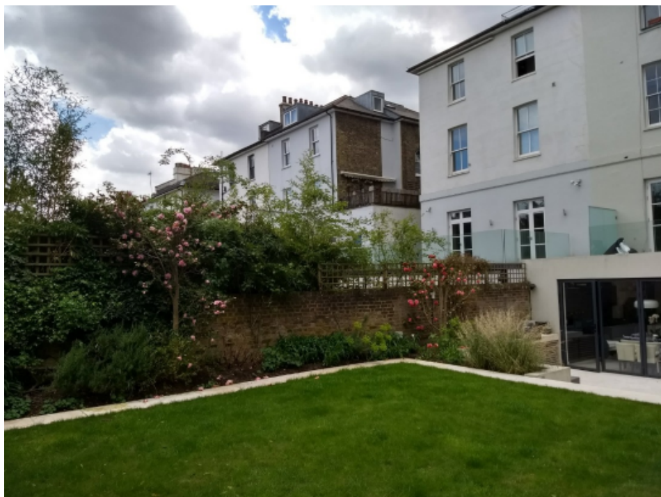
Photo 4: Boundary wall with 168 Haverstock Hill
