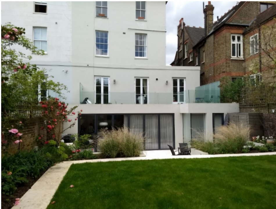
Photo 1: Rear elevation of 170 Haverstock Hill
