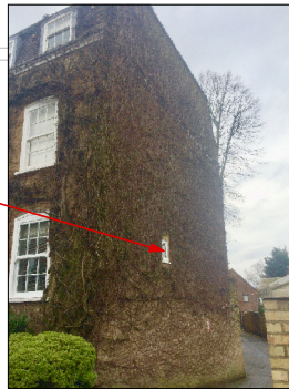
SIDE VIEW FROM NORTH END
