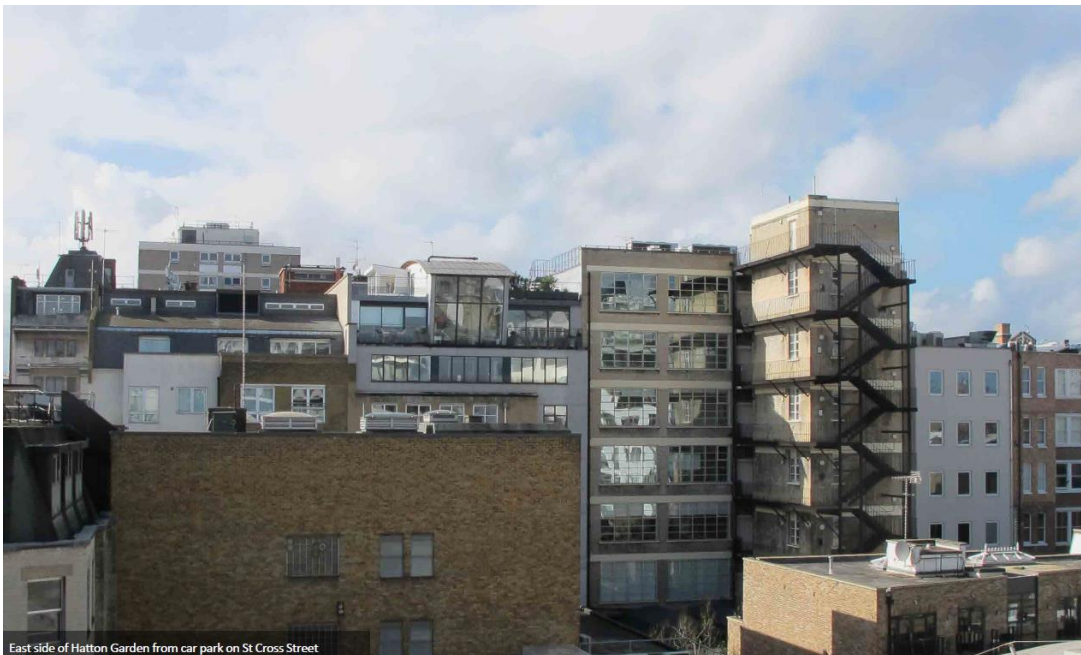
Above: Photograph taken from the Hatton Gardens Conservation Area Appraisal (2017)
