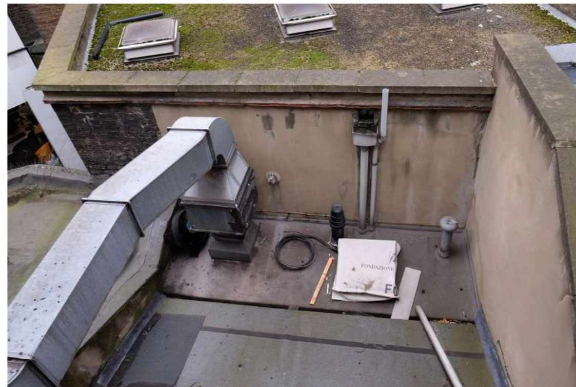
View looking out of rear window
