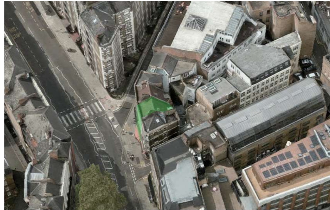
Aerial view looking West showing the site in green
