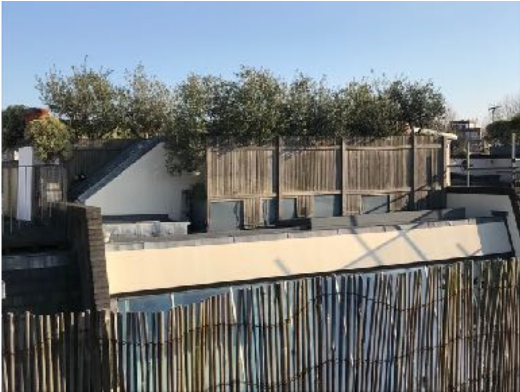
Image 7 Adjoining Buildings: Existing Roof Terrace Structures
