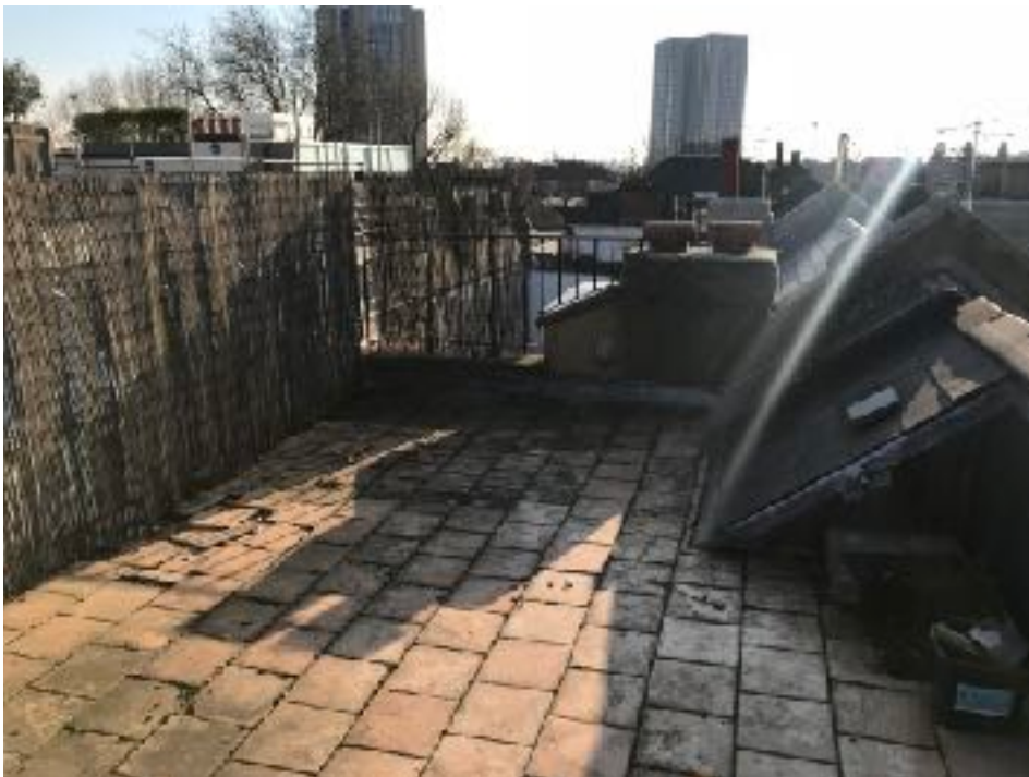
Image 6 Existing Roof Terrace Access
