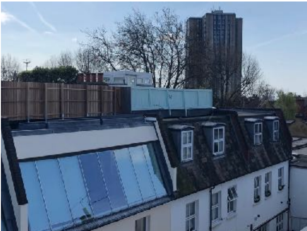
Image 8 Adjoining Buildings: Existing Roof Structures & Dormer Glazing
