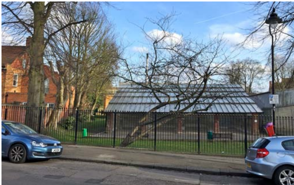
View towards the overall site from Broadlands Road: the trees are deciduous, but even in winter the Pool Hall building is barely visible, except for the tall boiler flue
