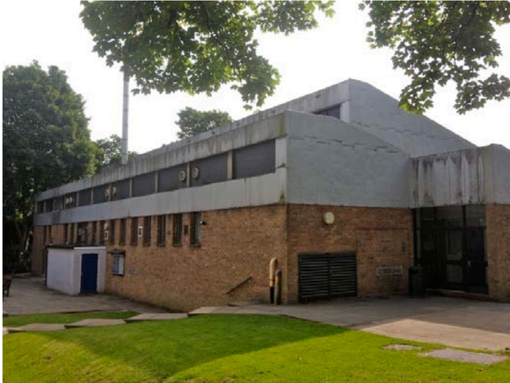
View of the north-west corner, with entrance to the right
