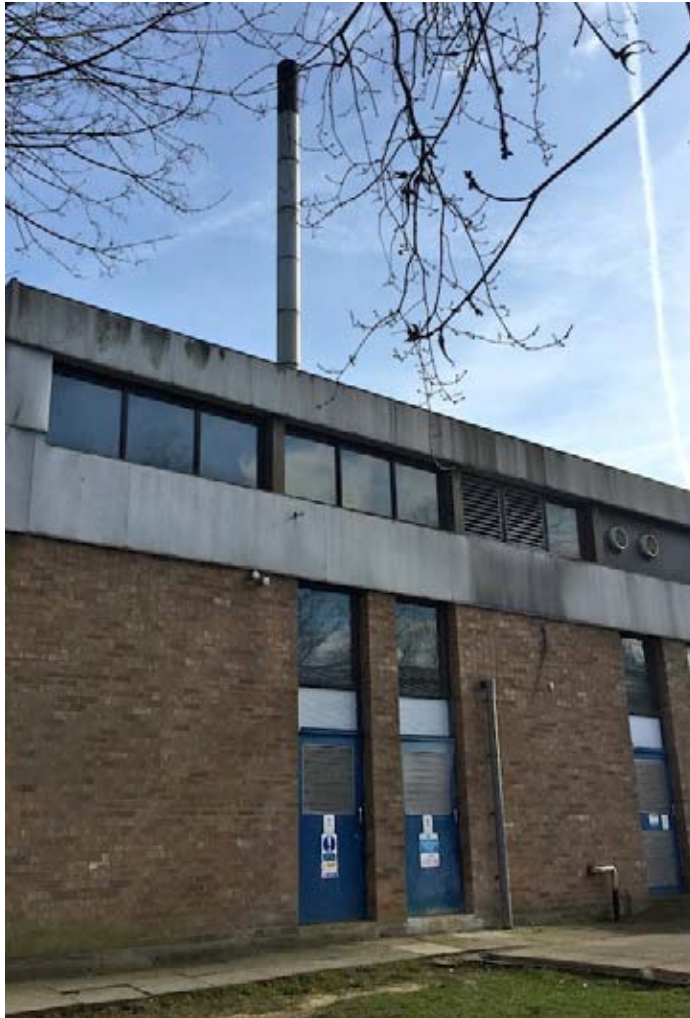
View of the north side of pool ancillary areas, with boiler flue
