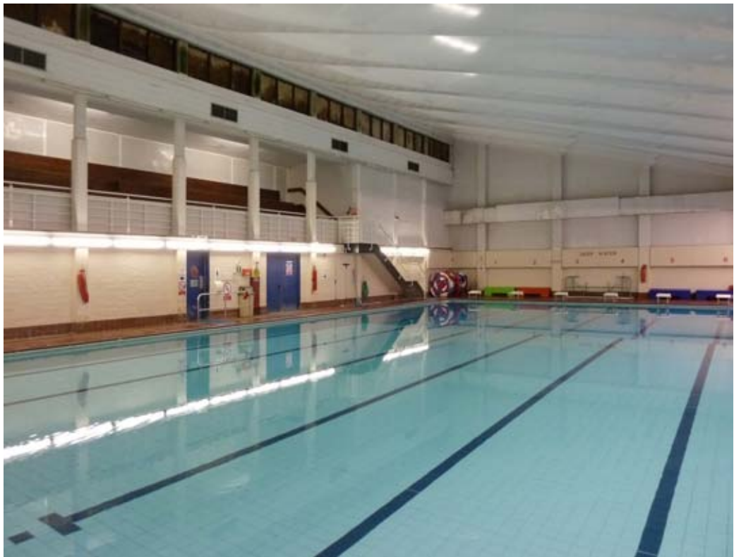
View of the pool hall interior at start of 2017, ceiling now removed, towards east end
