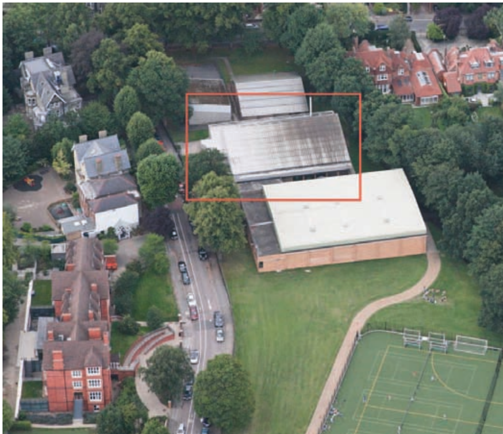
Aerial view of the MSC sports centre site from south, with pool hall behind sports hall
