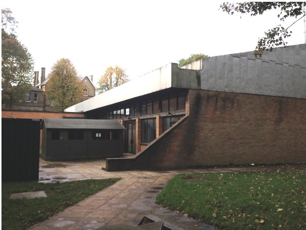
View of the pool hall from the south-east, with courtyard to the left
