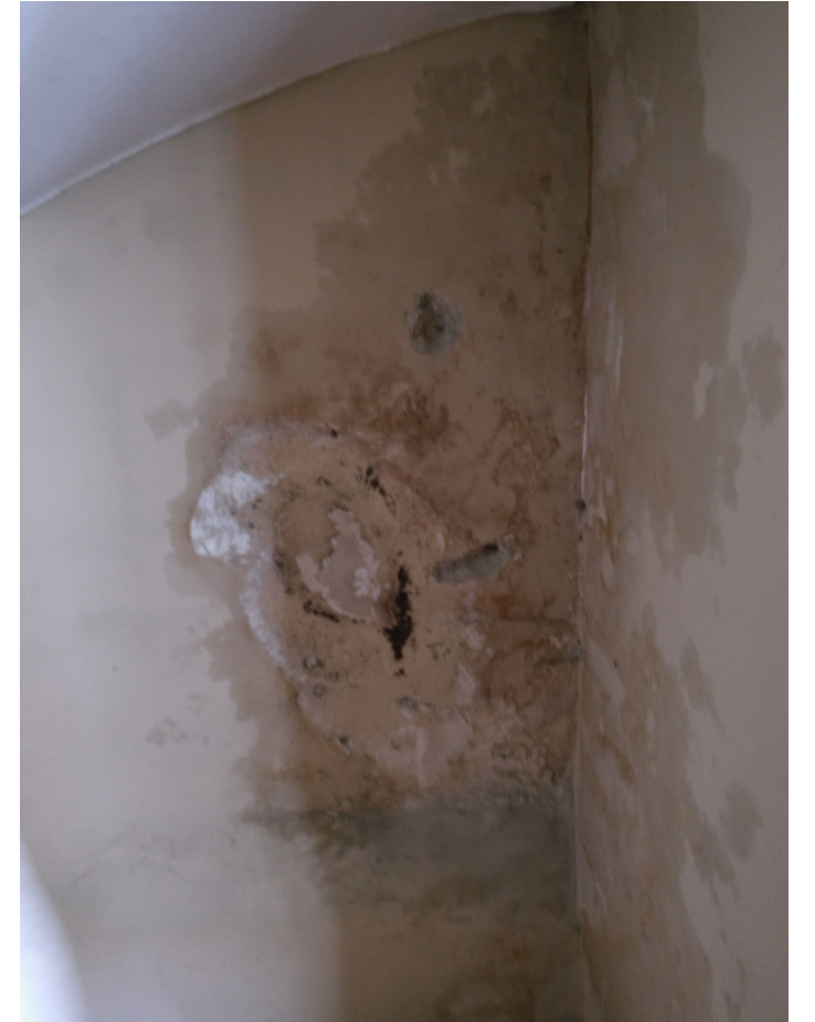
Internal water ingress
