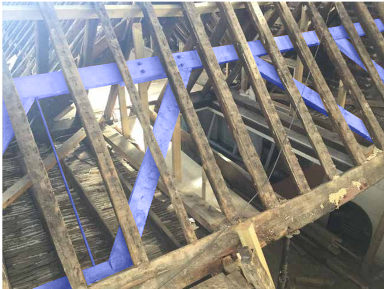
7 Denmark Street: Bracing in Front Roof Void
