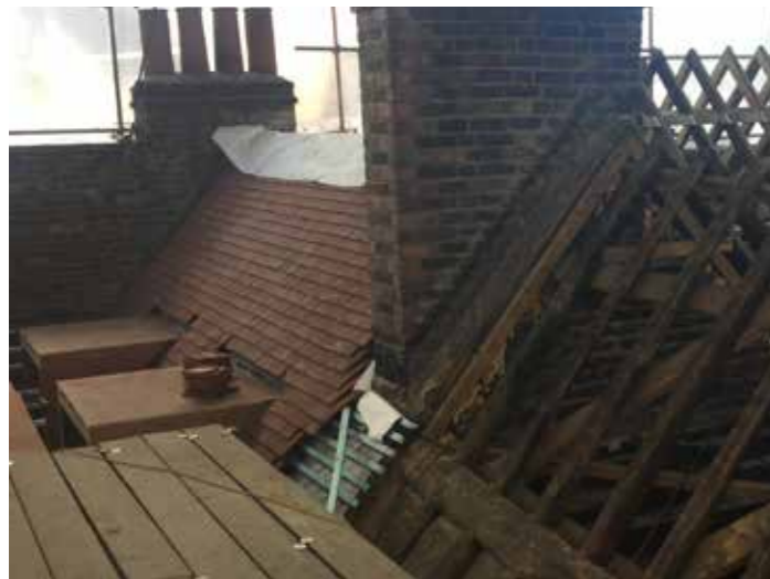
6 Denmark Street: Tiled Roof 7 Denmark Street: Exposed Structure
