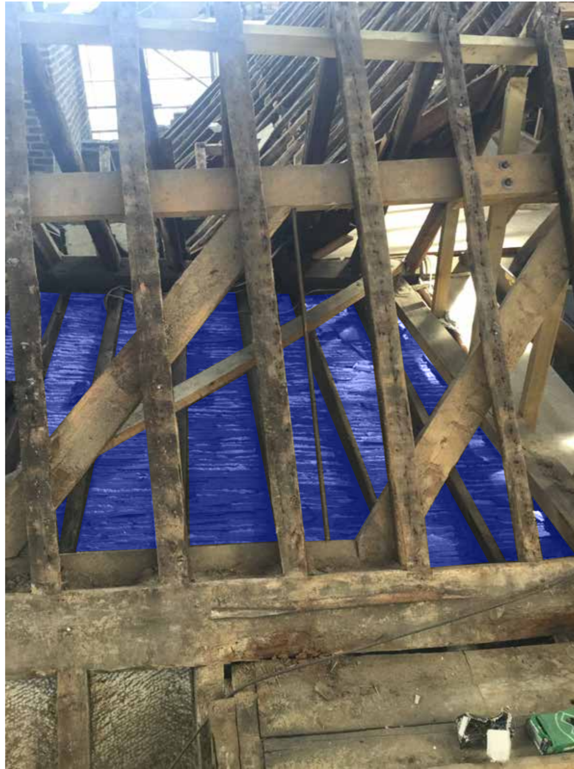
7 Denmark Street: Existing Ceiling Remains of existing lath and plaster ceilings
