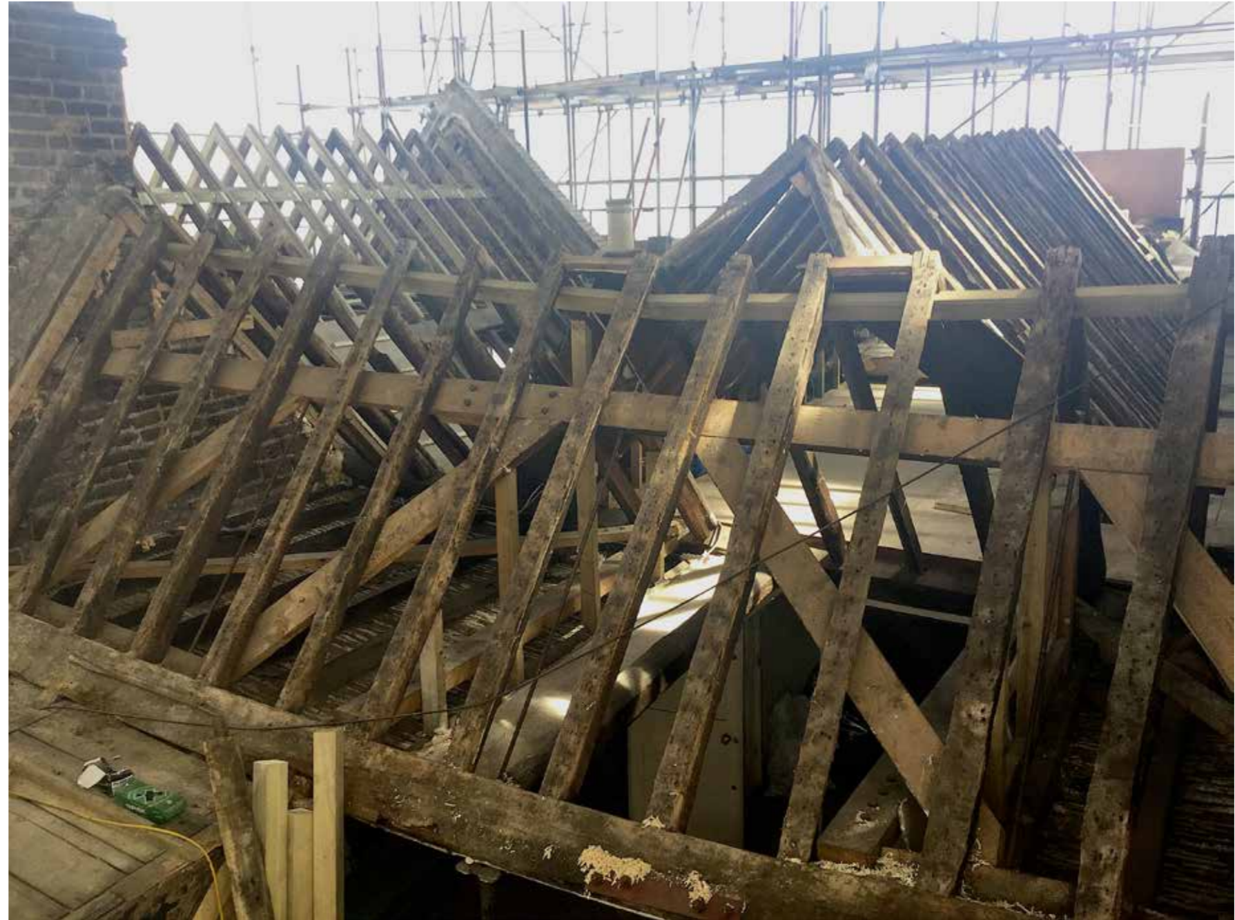
7 Denmark Street: Front Roof Pitch
