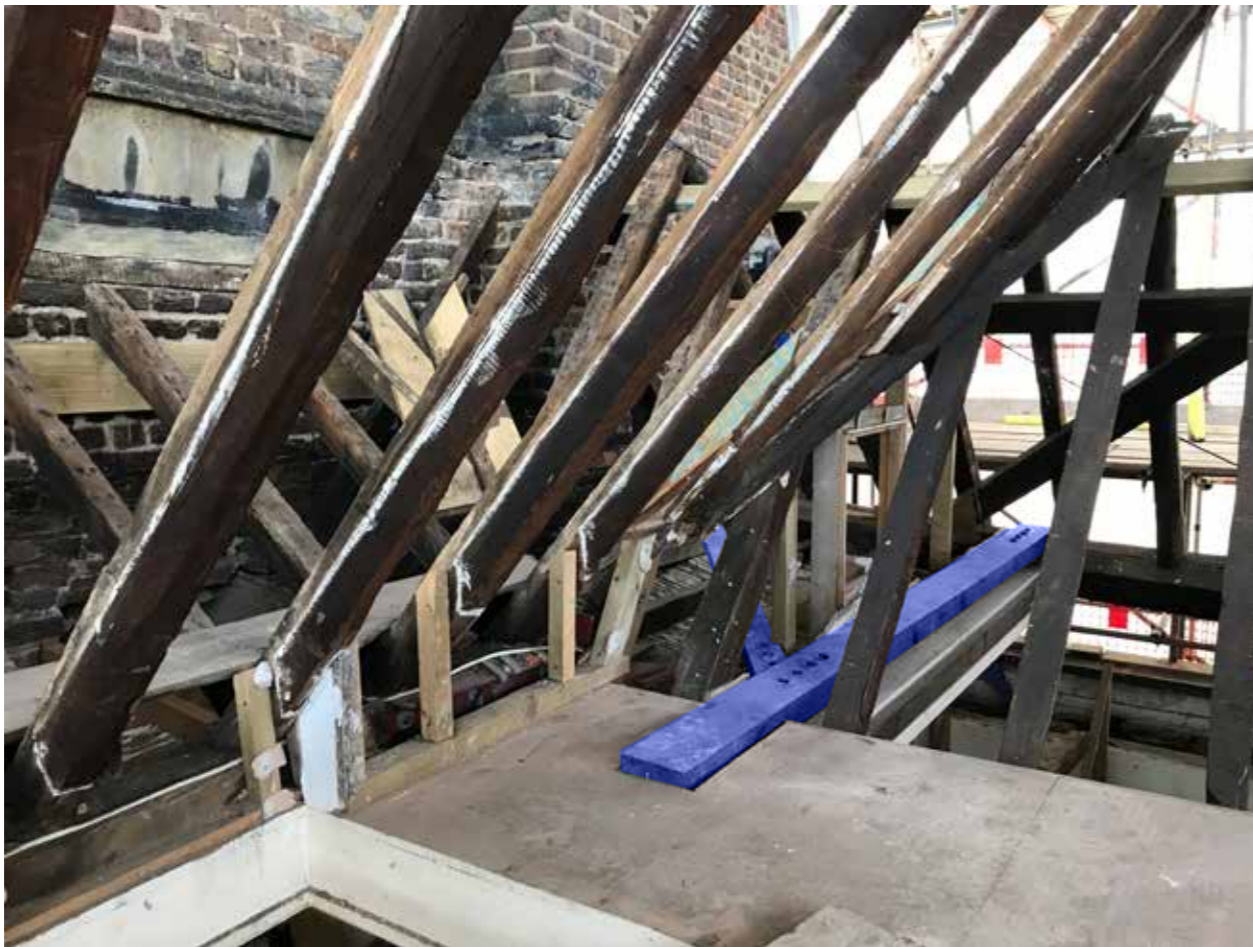
7 Denmark Street: Bracing Around Ceiling Opening
