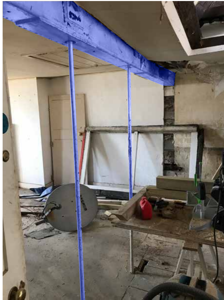
7 Denmark Street: Steel Supports
