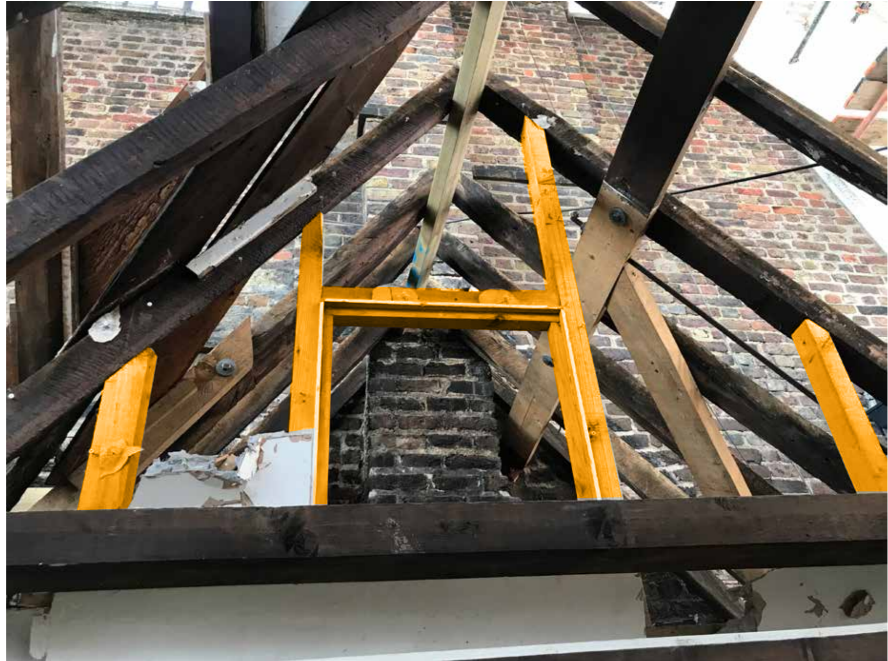
7 Denmark Street: 20th Century Timber Struts in Roof Void
