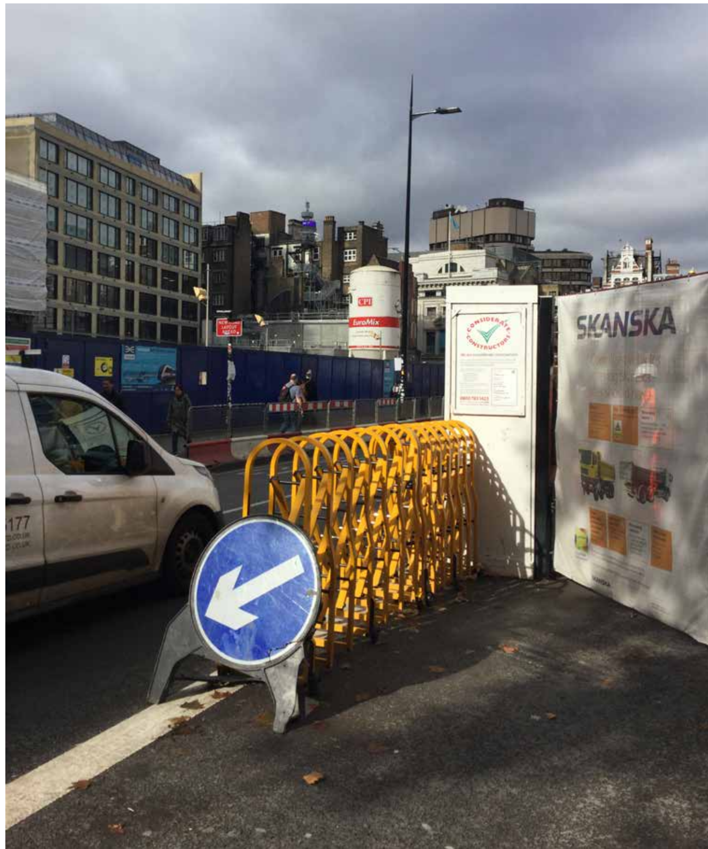
Examples of the of style of hoarding, bi-fold entrance gates, signage, retractable barriers and traffic controllers proposed - seen at a neighbouring site along Charing Cross Road
