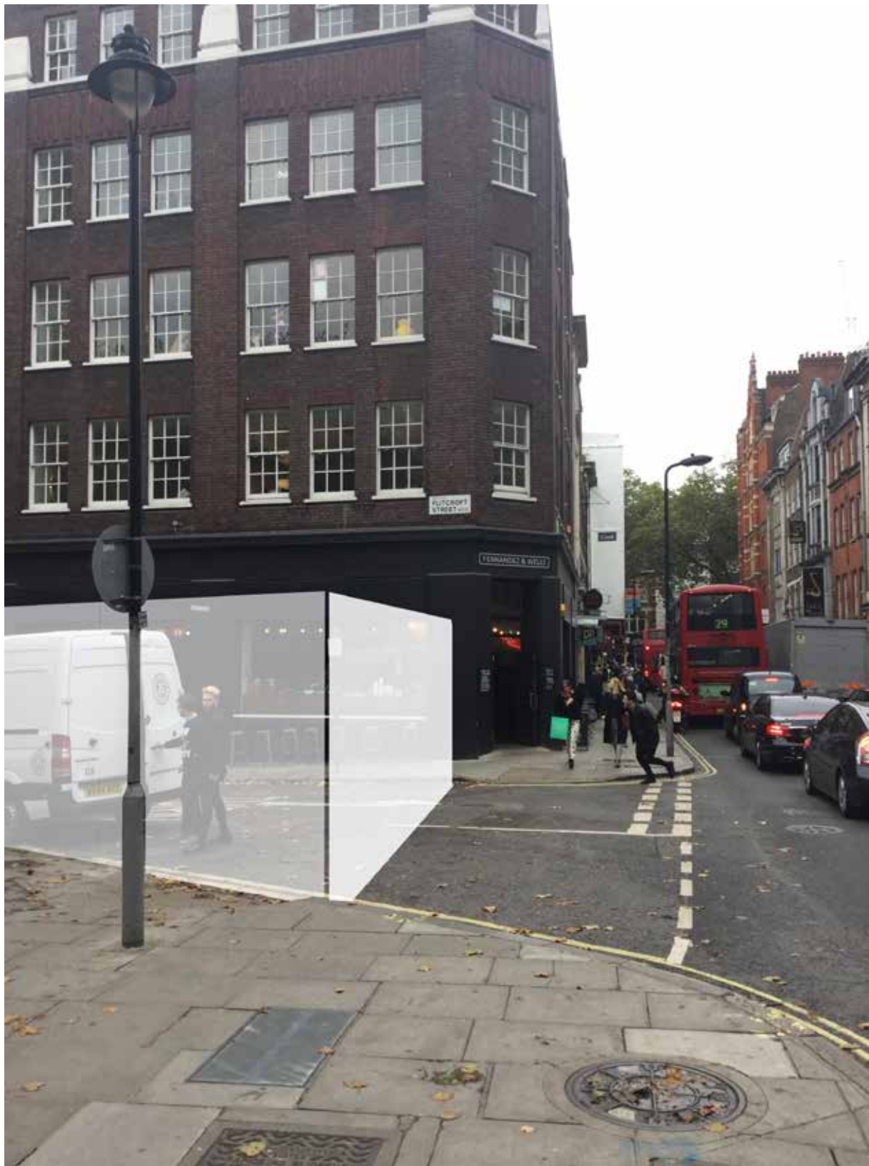
Hoarding set back from the building line of Denmark Street, providing uninterrupted views along the street from St Giles High Street, and providing access to the ground level retail spaces
