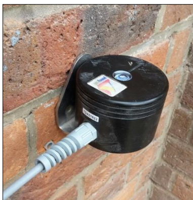
Example of Vibration Unit installation on wall
