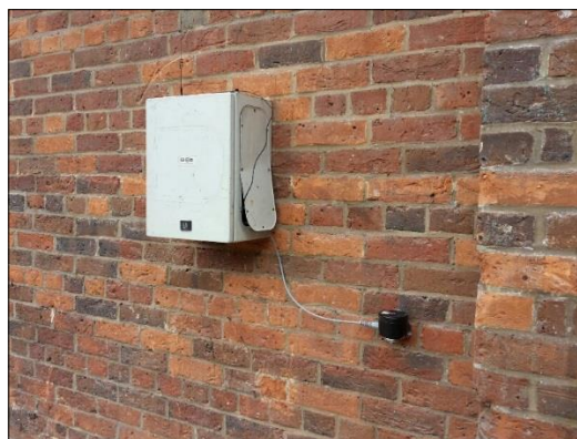
Example of Vibration Unit installation on wall
