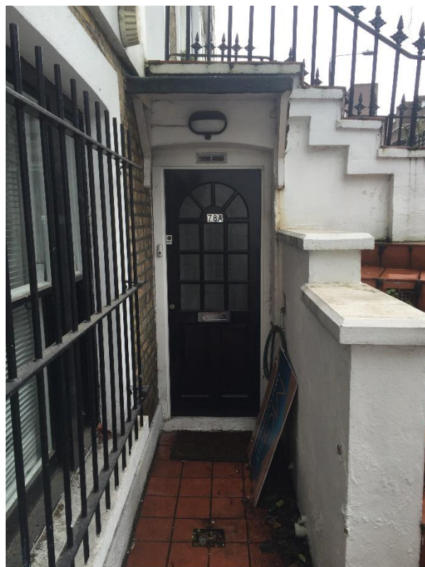
Existing entrance to lower ground floor level
