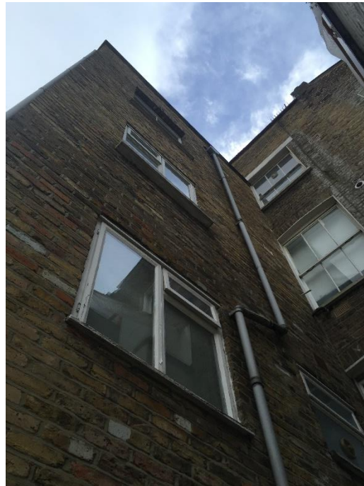
Existing Rear extension
