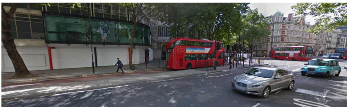
Figure 5 Setting of listed buildings at the appeal site (Google)
