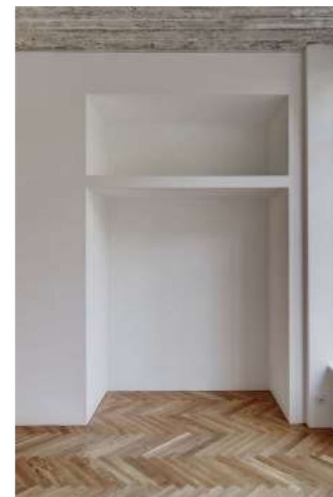
New partitions are to be read separately from the existing building, by use of plain, painted plasterboard walls
