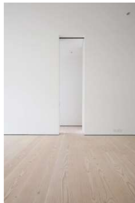
Shadow gaps will be used on all new partitions at every junction with the existing building fabric, following exact profiles
