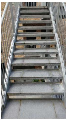
The two flights are 6 and 11 steps instead of 9 and 9. The finish is uncoated galvanised steel. Safety rods not in evidence.
