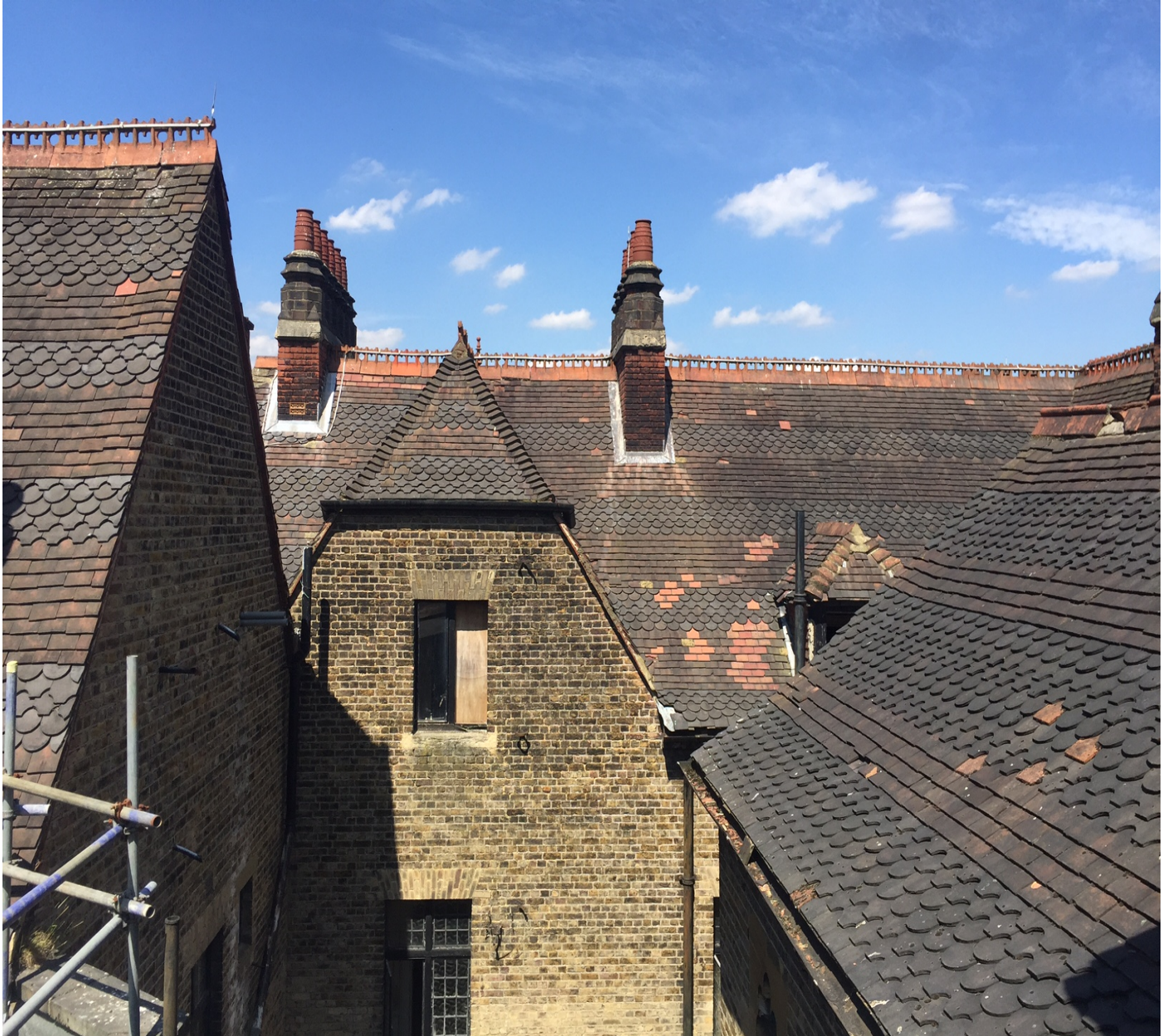
PHOTOS 3 OF 6 NOMINATED ROOF AREA
