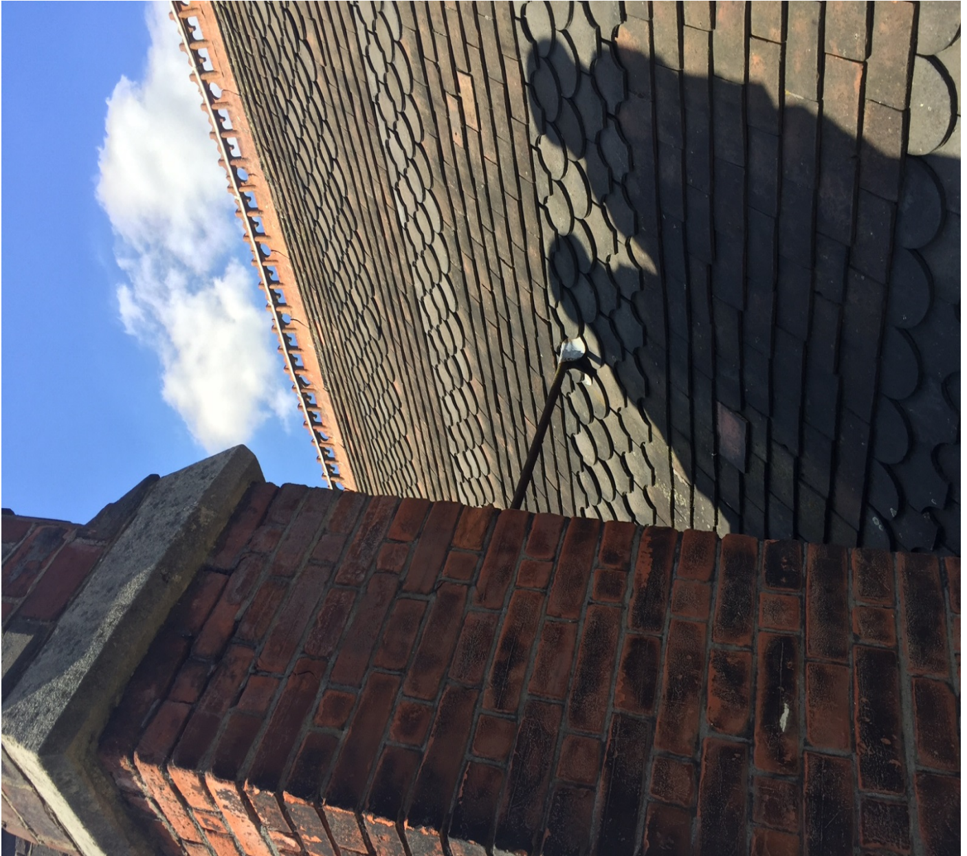
PHOTOS 6 OF 6 NOMINATED ROOF AREA
