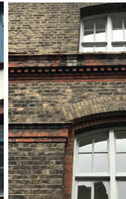
EXISTING MATERIALITY OF ADJACENT 3 FLITCROFT ST ASSUMED TO MATCH THE ORIGINAL MATERIALITY OF 4 FLITCROFT ST.
