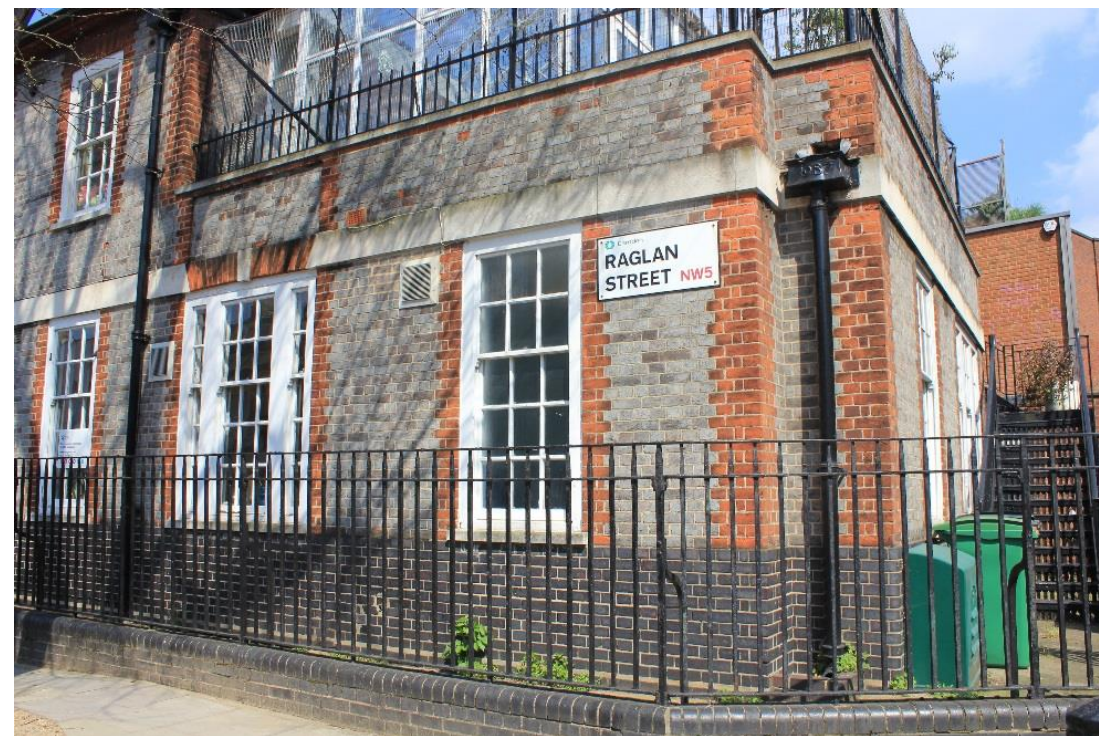
THE RAGLAN HOUSE DAYCARE CENTRE ACROSS FROM SITE
