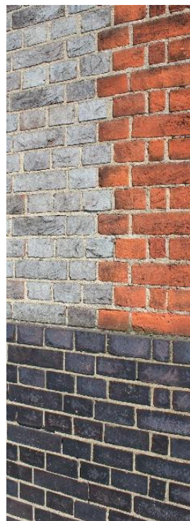
CLOSE UP OF BRICKWORK
