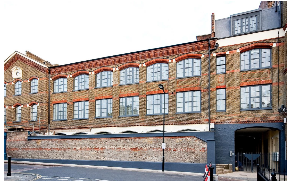
REFURBISHMENT (5-8 Anglers Lane)
