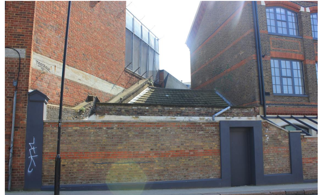
EXISTING FRONT ELEVATION (5 Anglers Lane) – The rear of 1-2 Anglers Lane can be seen at street level due to the low composition of the current building, spoiling the views within the Inkerman Conservation Area
