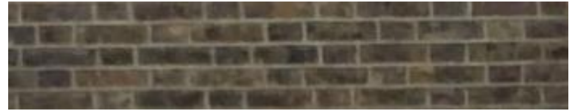
EXISTING AGED BRICKWORK (5-8 Anglers Lane)
